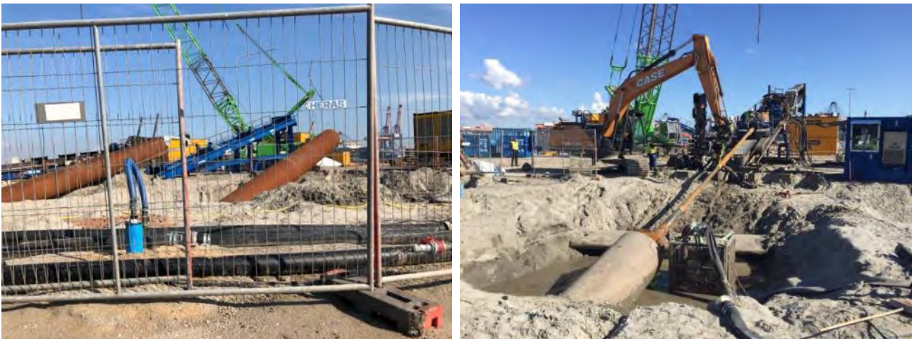
Figure 25 - Examples of reamer in HDDs
