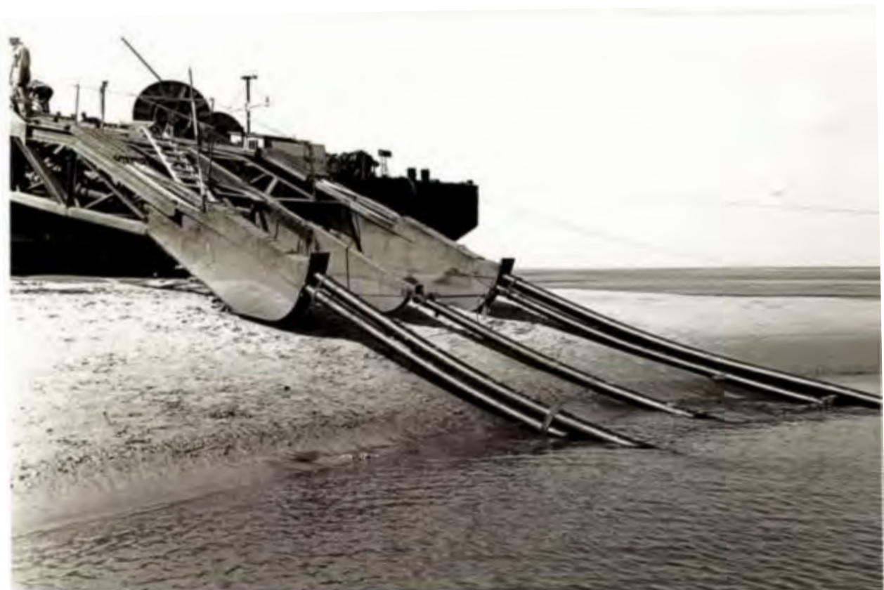
Figure 52 Detail of the barge mounted Vertical Injector like trencher in Zeeland
