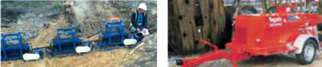
Figure 18 Typical cable tensioners (left) & cable winch (right)
