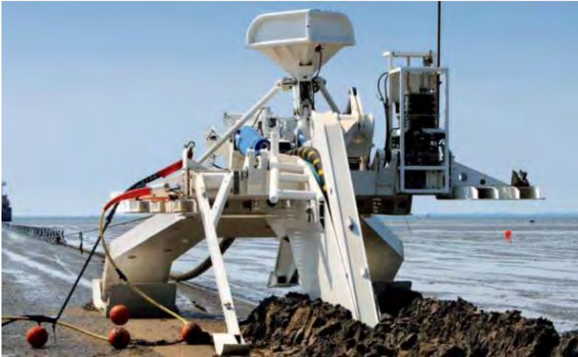
Figure 45 Sea Stallion cable plough
