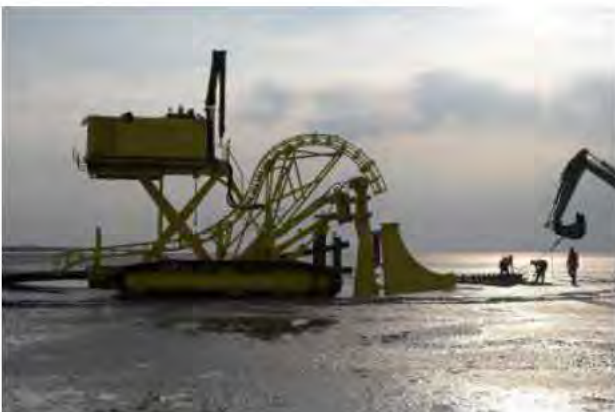
Figure 54 Vibration plough on tracks
