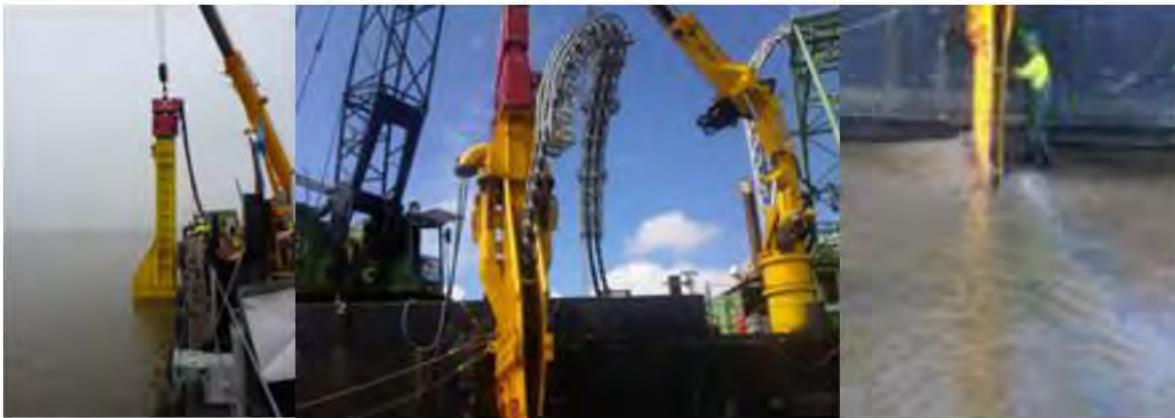
Figure 53 Vibration plough deployed from a barge
