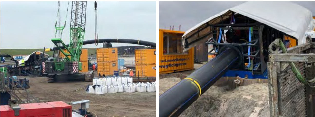
Figure 118 Pipe string supply into pipe pusher
