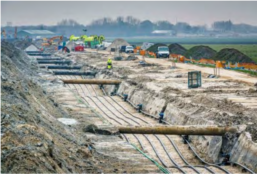
Figure 15 Example of a trench
