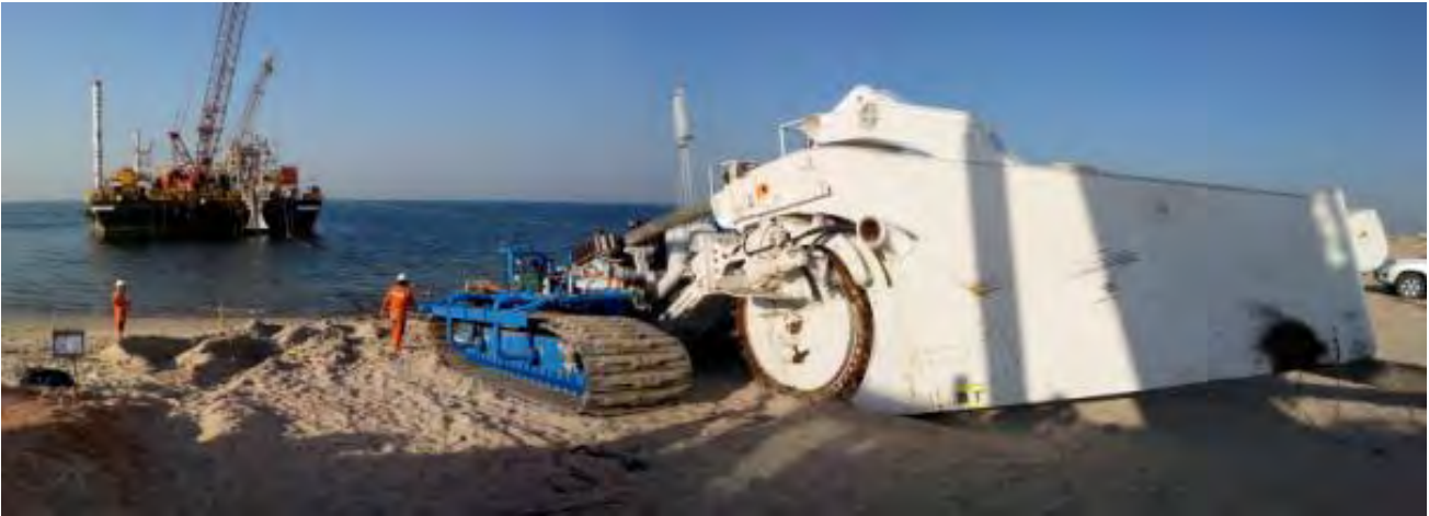
Figure 44 TM04 Wheel cutter cable trencher
