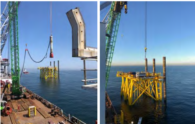
Figure 6 Pile driving at Borssele Alpha
