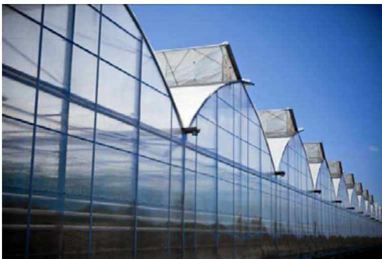
Photo: double sided butterfly ventilation system
