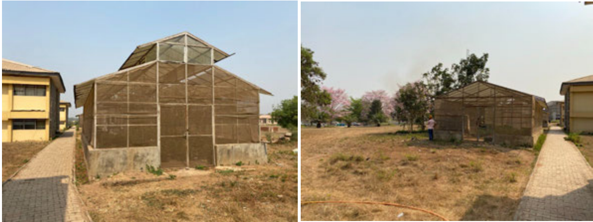
Photo Local constructed, low costs and simple small green houses in Nigeria
