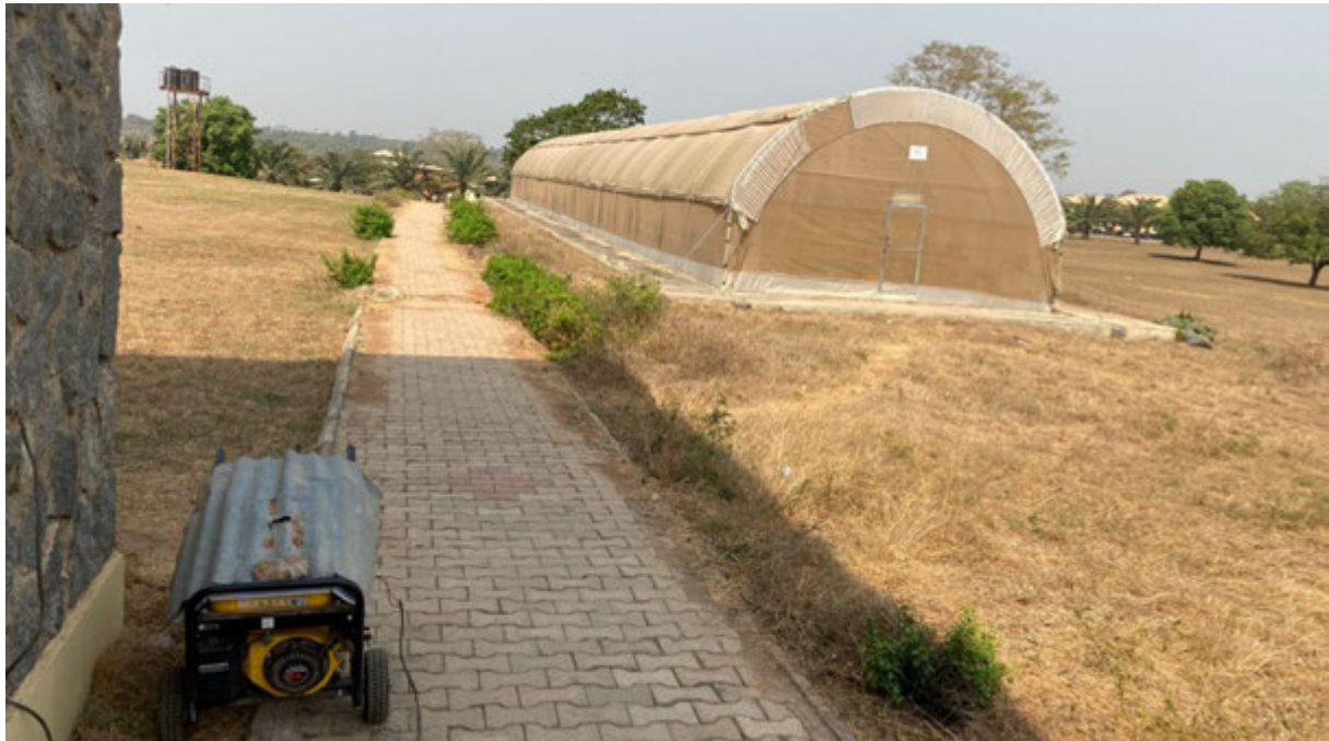
Photo low tech single span greenhouse 1
