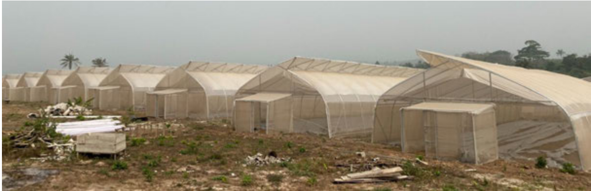
Photo: Single span single side butterfly ventilation green house in South West Nigeria
