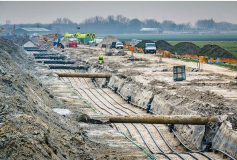
Figure 15 Example of a trench
