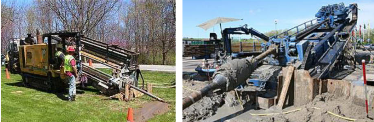
Figure 32 Example HDD rigs - [left] midi rig - [right] maxi rig
