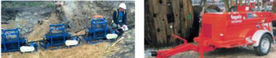
Figure 18 Typical cable tensioners (left) & cable winch (right)
