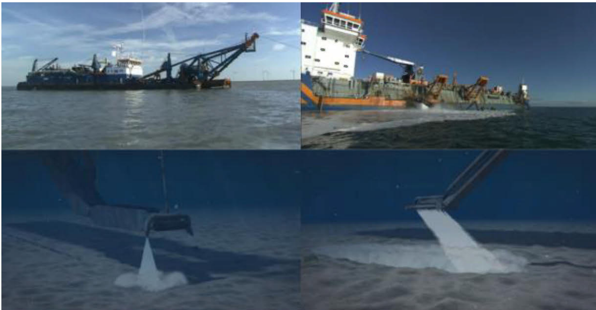
Figure 47 Mass flow excavation by a converted Suction Dredger or Hopper Dredger
