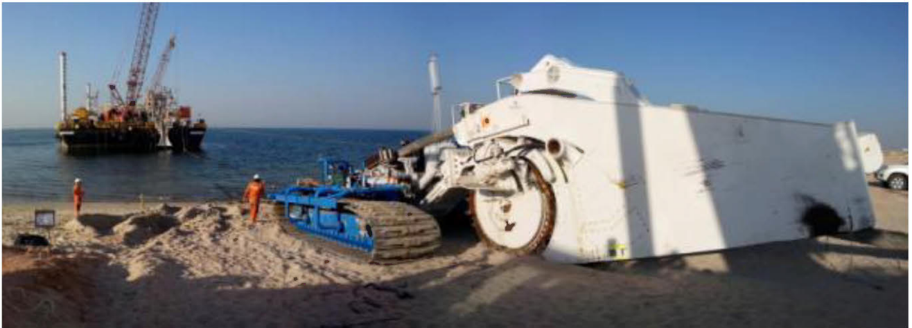
Figure 44 TM04 Wheel cutter cable trencher
