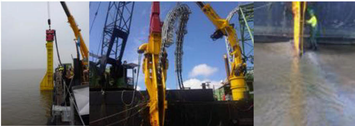
Figure 53 Vibration plough deployed from a barge
