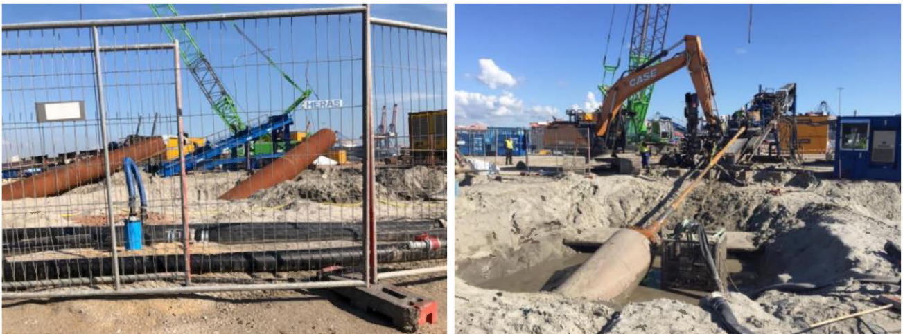
Figure 25 - Examples of reamer in HDDs
