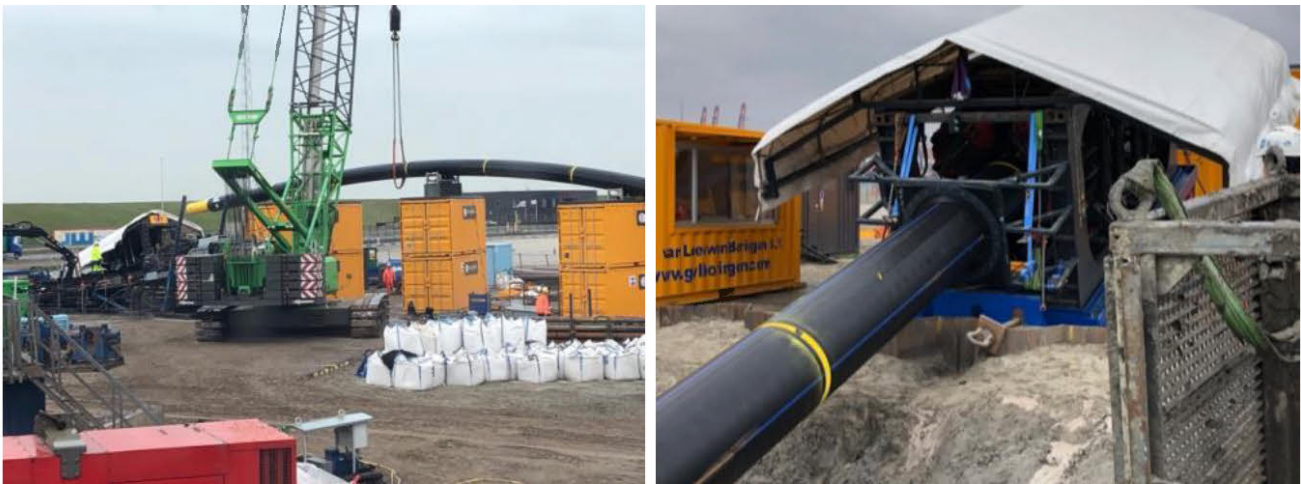
Figure 118 Pipe string supply into pipe pusher
