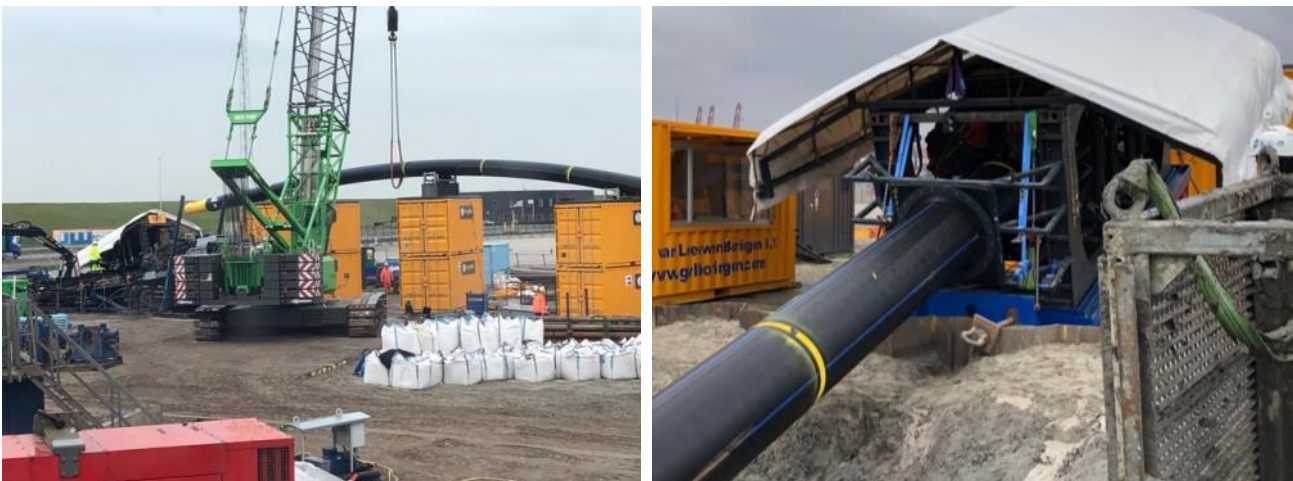
Figure 118 Pipe string supply into pipe pusher
