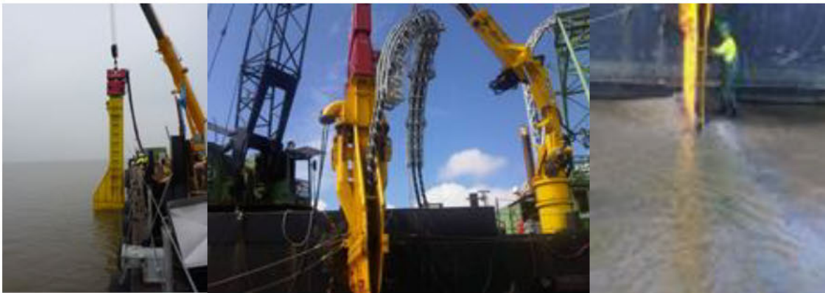
Figure 53 Vibration plough deployed from a barge
