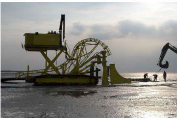
Figure 54 Vibration plough on tracks
