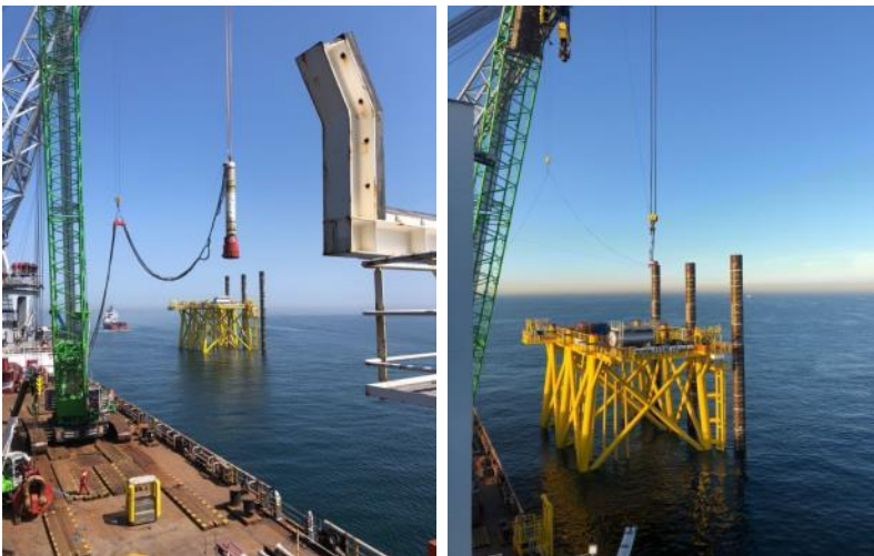
Figure 6 Pile driving at Borssele Alpha
