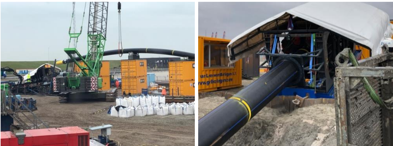
Figure 118 Pipe string supply into pipe pusher
