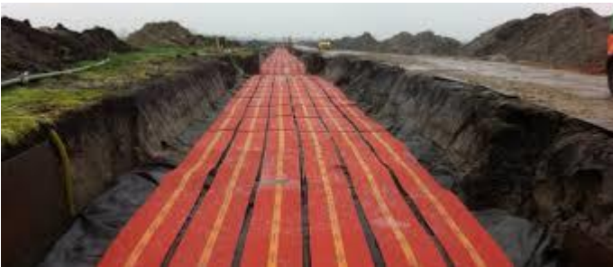
Figure 19 Open cable trench, after the pull-in of the cables
