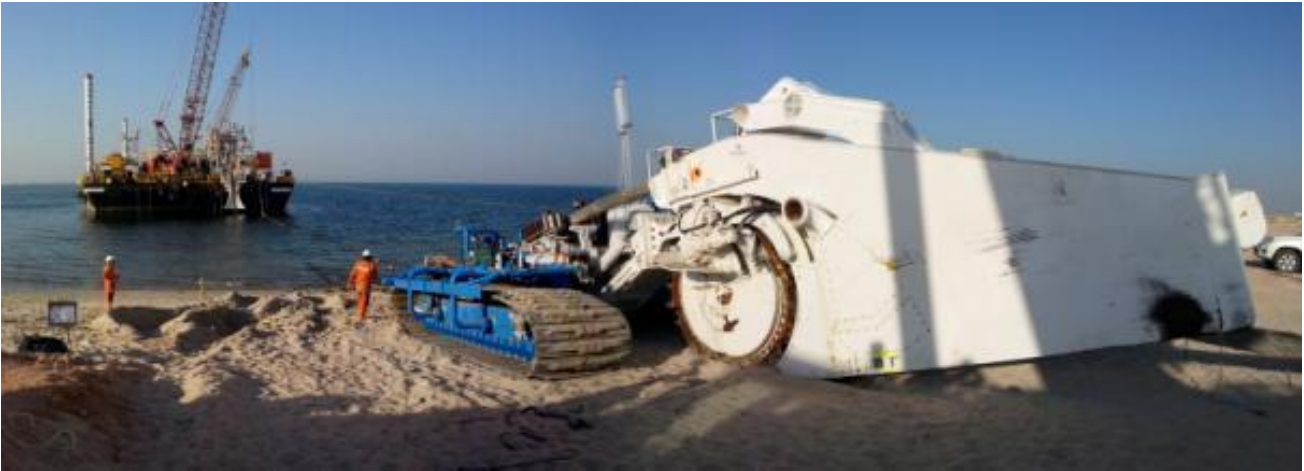
Figure 44 TM04 Wheel cutter cable trencher
