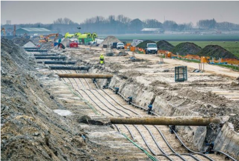
Figure 15 Example of a trench
