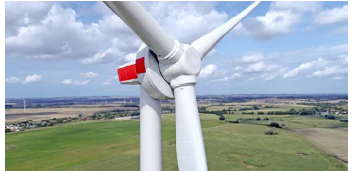
HYGRO specialises in the production, delivery and distribution of hydrogen produced directly from wind. It is building a 4-MW wind turbine with an integrated electrolyser in the province of North Holland. The aim is to maximise synergy between wind power, hydrogen and pipeline & storage technology. The concept optimises conversion of wind power to hydrogen, which can be transported at much lower cost than electricity and with a significantly lower impact on spatial planning.
