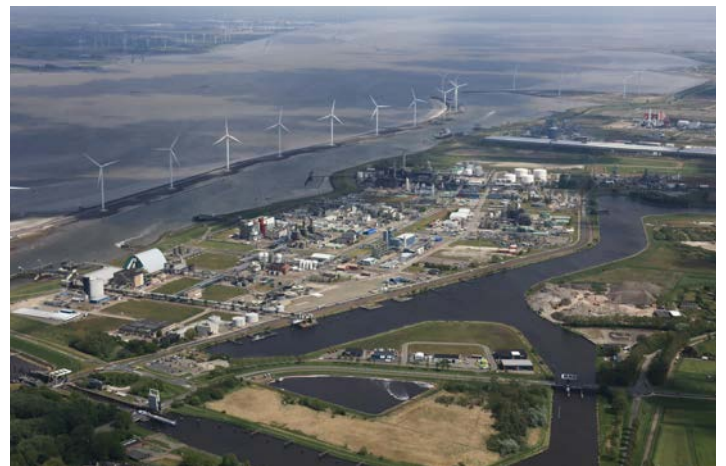
In the northern coastal town of Delfzijl, gas grid operator Gasunie and HyCC are planning to build a 20-MW electrolyser, which will produce 3,000 tonnes of clean hydrogen each year. They are also studying options to expand its capacity to 60 MW in order to produce sustainable jet fuel. (Photo: Groningen Seaports/Koos Boertjens)
