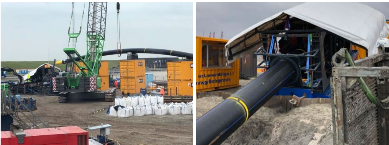
Figure 26 Pipe string supply into pipe pusher
