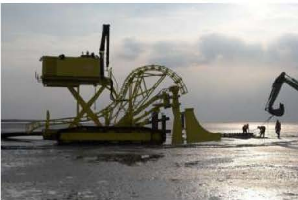
Figure 52 Vibration plough on tracks
