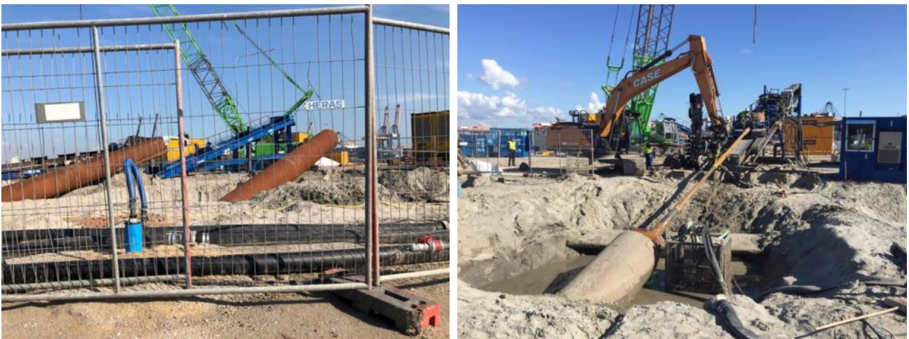
Figure 23 - Examples of reamer in HDDs
