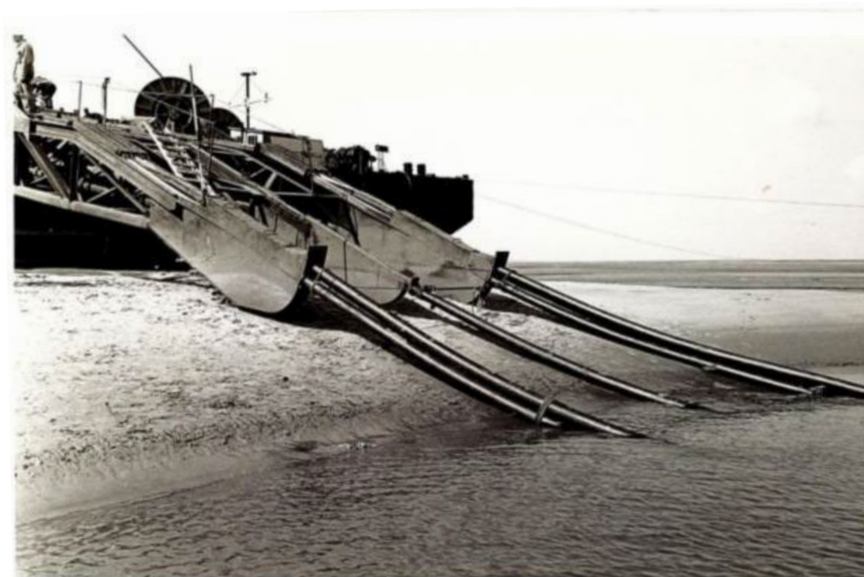
Figure 50 Detail of the barge mounted Vertical Injector like trencher in Zeeland
