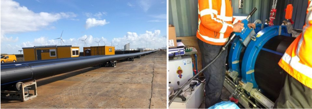
Figure 25 Pipe string assembly and mirror welding technique in container.
