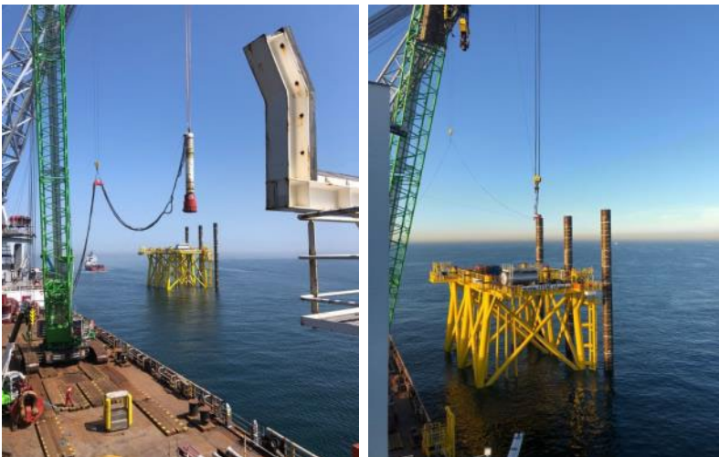
Figure 6 Pile driving at Borssele Alpha
