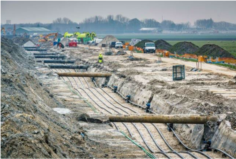
Figure 13 Example of a trench
