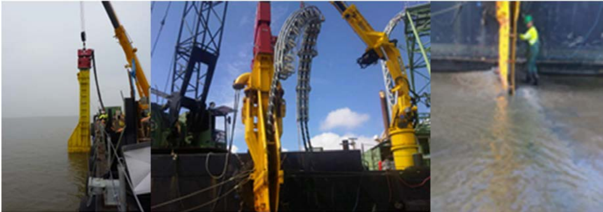
Figure 50 Vibration plough deployed from a barge
