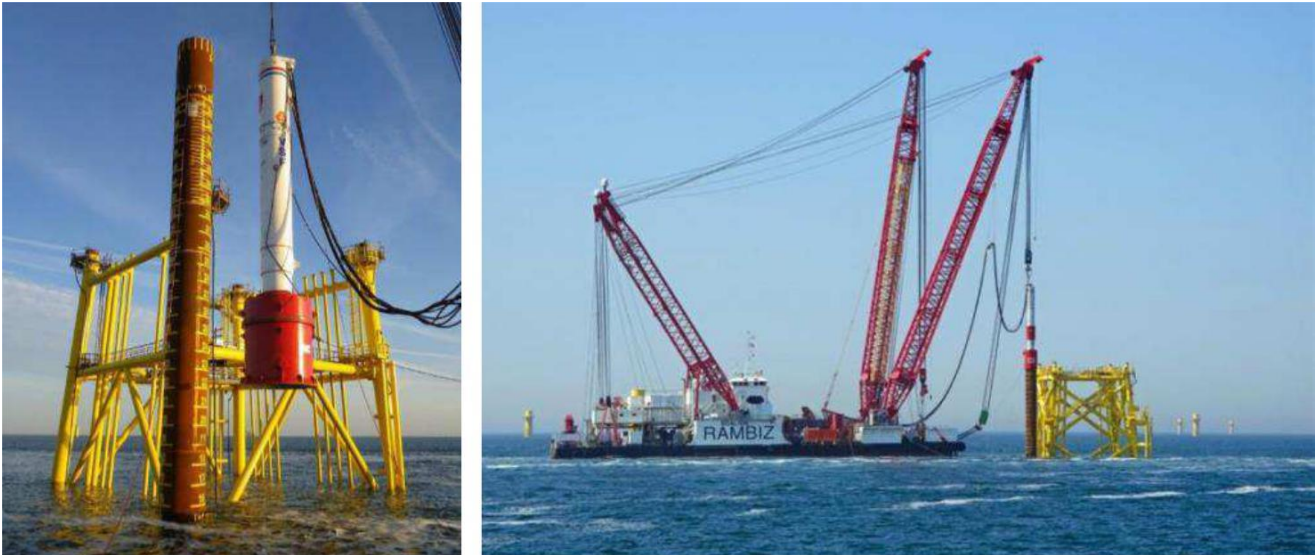
Figure 59 Piling of jacket
