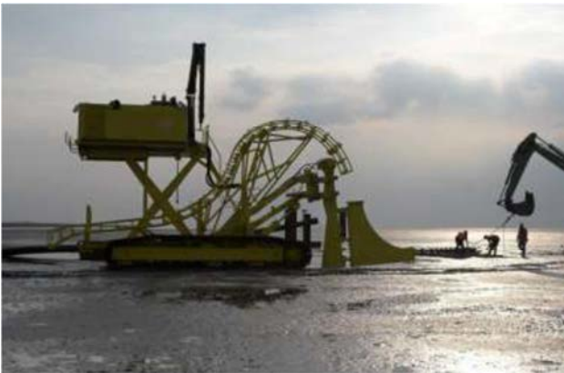
Figure 51 Vibration plough on tracks
