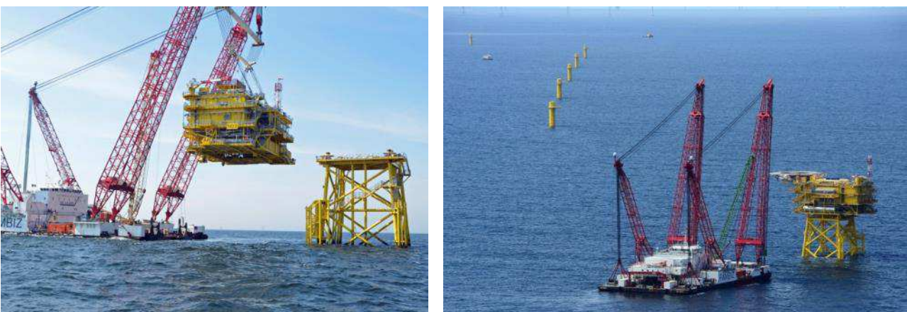
Figure 60 Installation of topside
