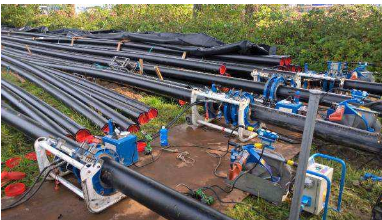
Figure 27 Welding of HDPE ducts
