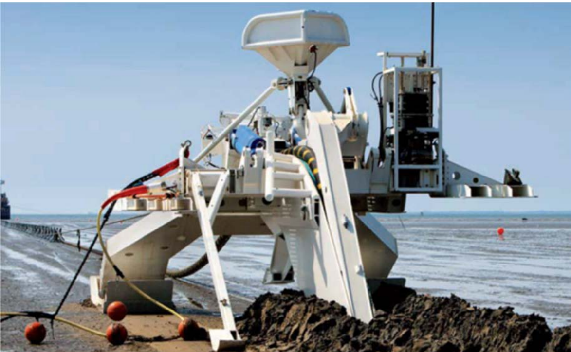
Figure 42 Sea Stallion cable plough
