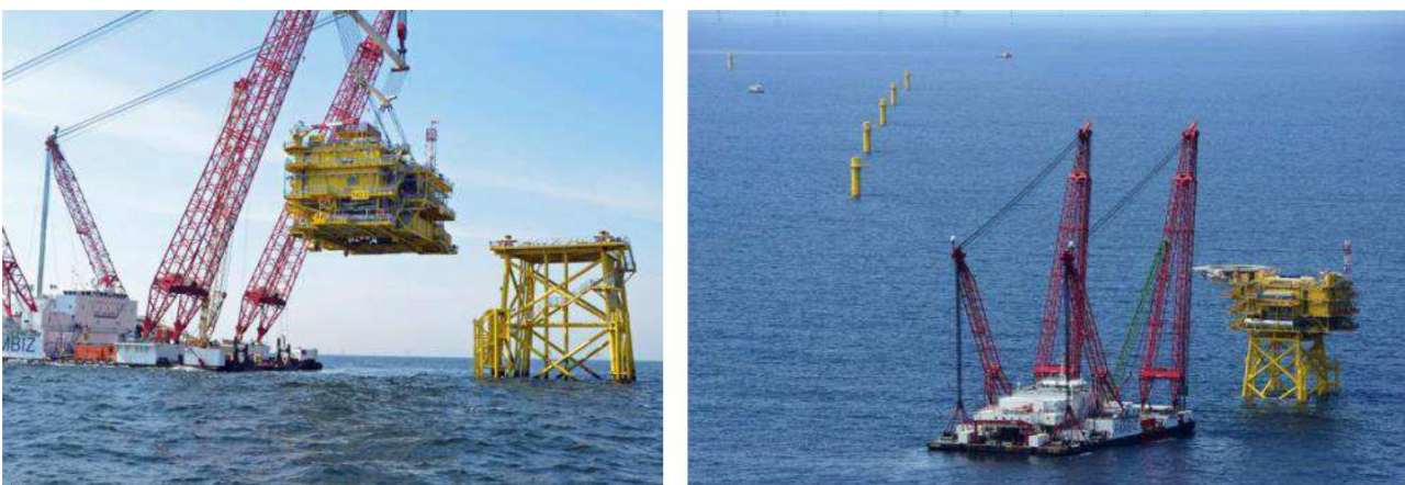
Figure 60 Installation of topside
