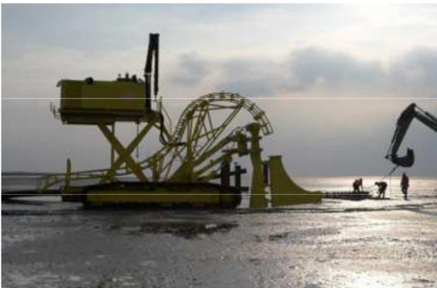
Figure 51 Vibration plough on tracks
