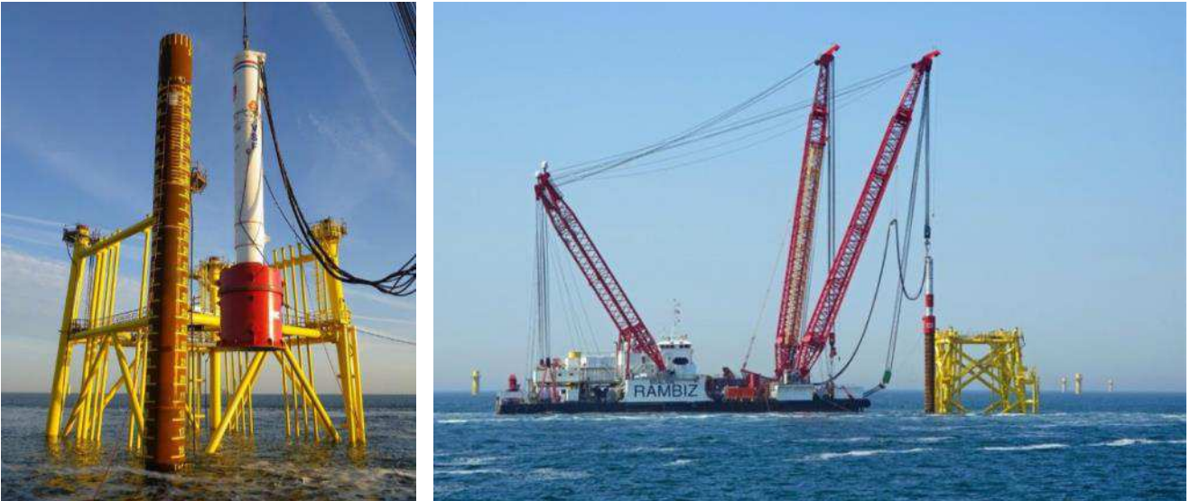
Figure 59 Piling of jacket
