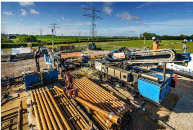
Figure 26 Example of HDD entry and exit point
