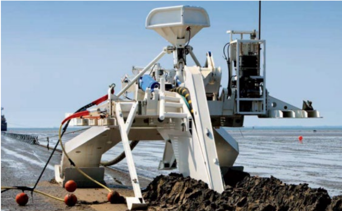
Figure 43 Sea Stallion cable plough
