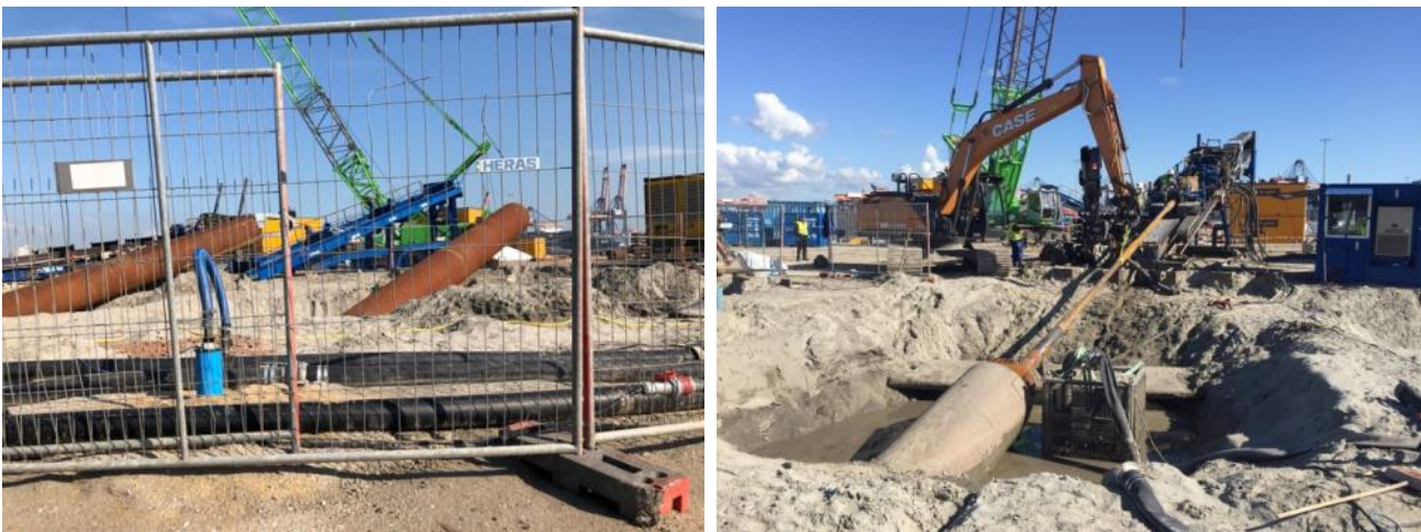
Figure 23 - Examples of reamer in HDDs
