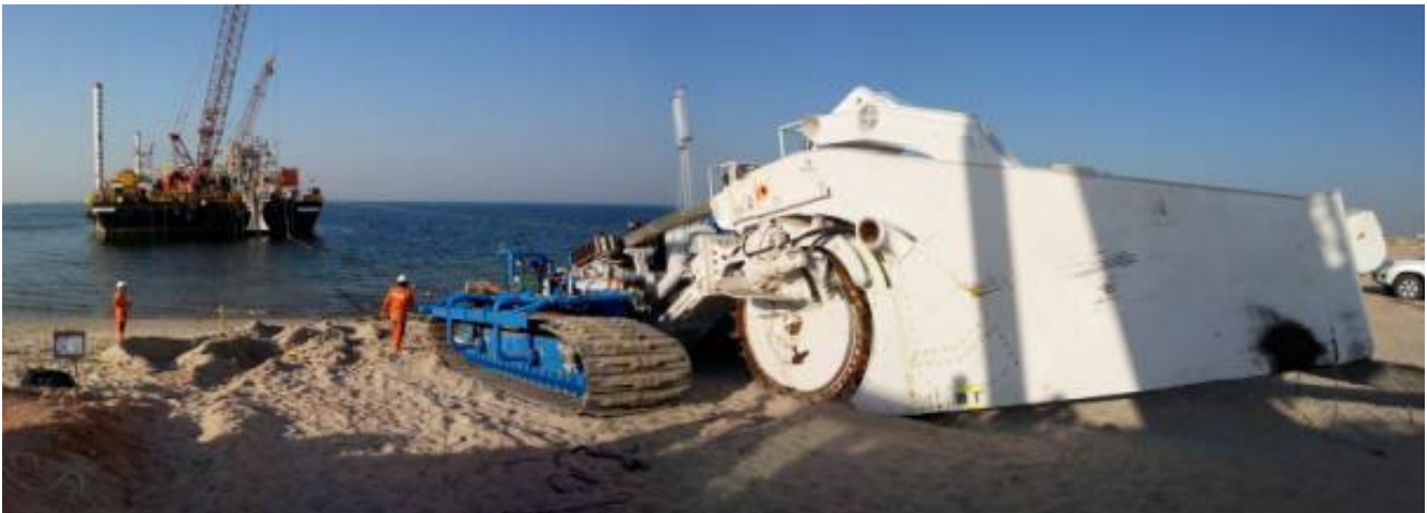
Figure 42 TM04 Wheel cutter cable trencher
