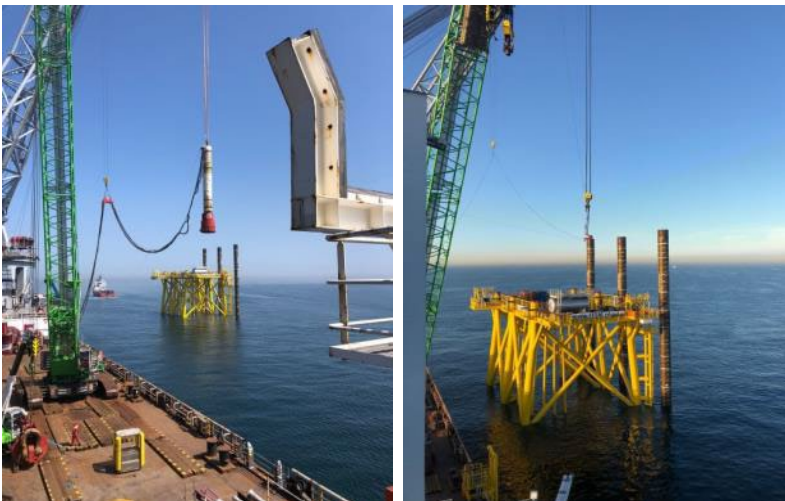
Figure 6 Pile driving at Borssele Alpha
