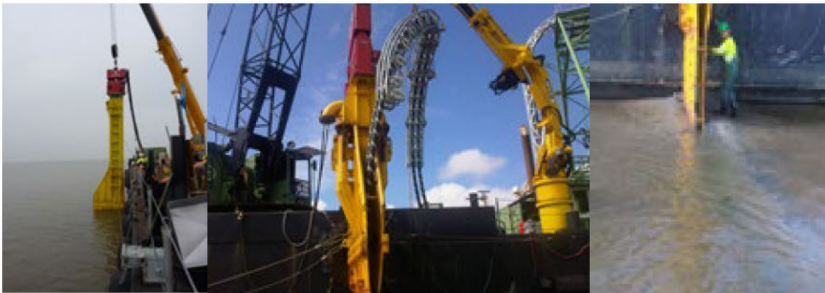
Figure 51 Vibration plough deployed from a barge
