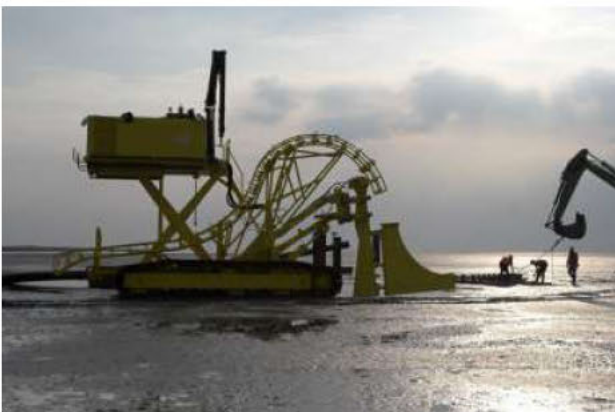
Figure 52 Vibration plough on tracks
