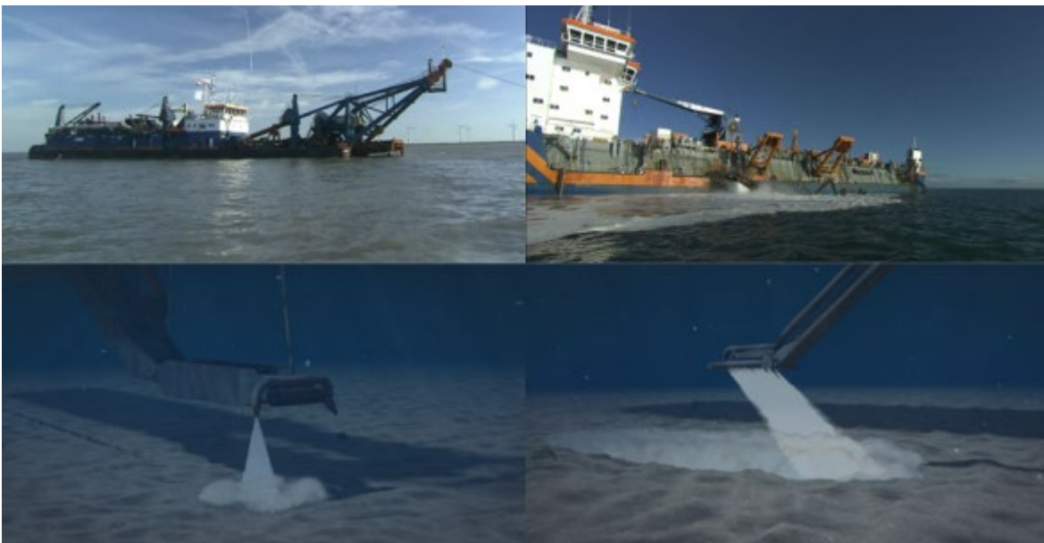
Figure 45 Mass flow excavation by a converted Suction Dredger or Hopper Dredger
