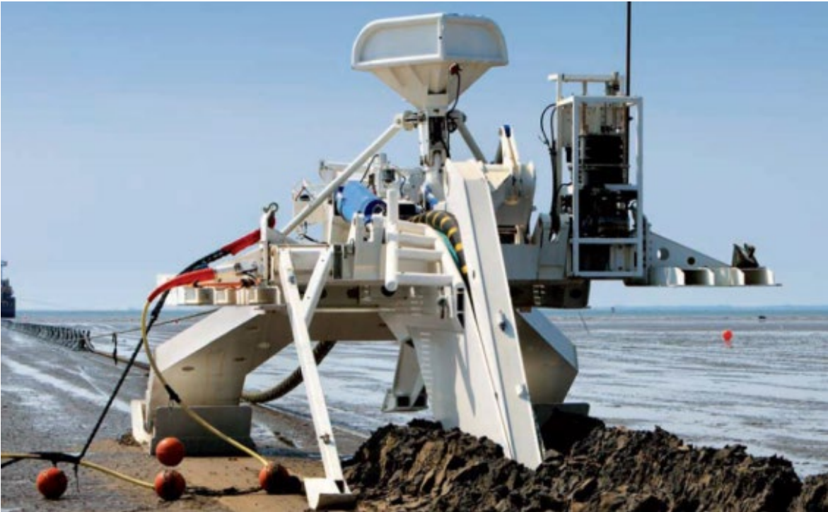
Figure 43 Sea Stallion cable plough
