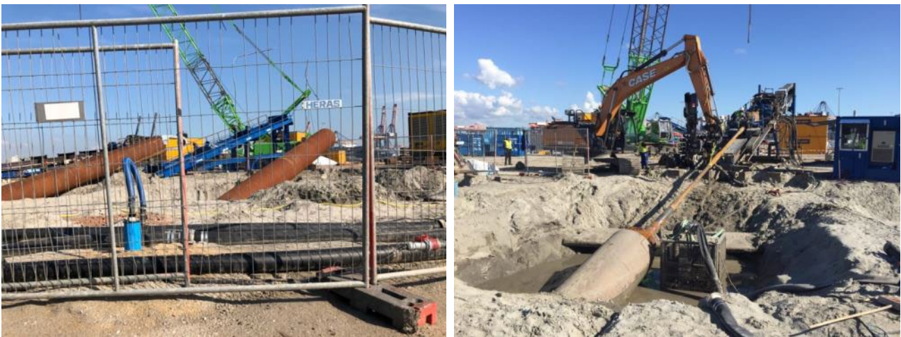
Figure 23 - Examples of reamer in HDDs
