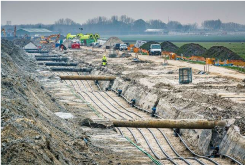
Figure 13 Example of a trench
