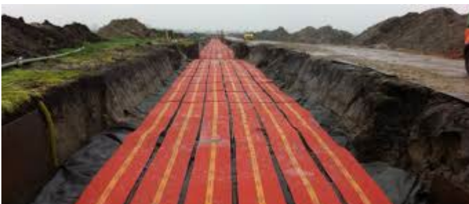
Figure 17 Open cable trench, after the pull-in of the cables
