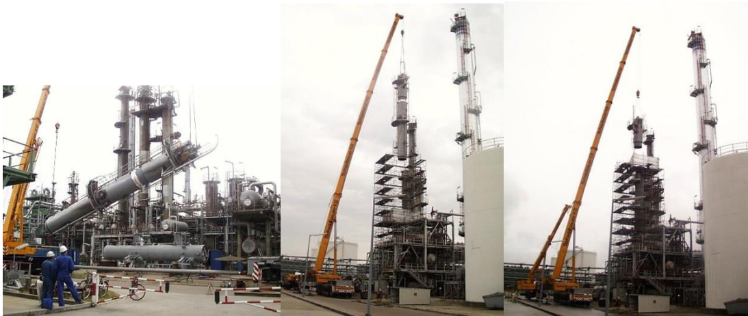
Installation of column on site
