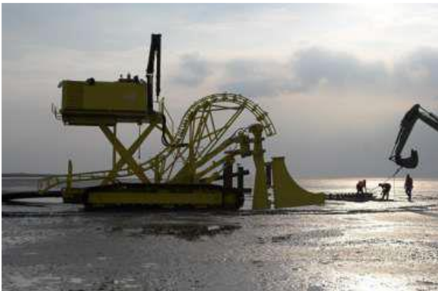
Figure 54 Vibration plough on tracks
