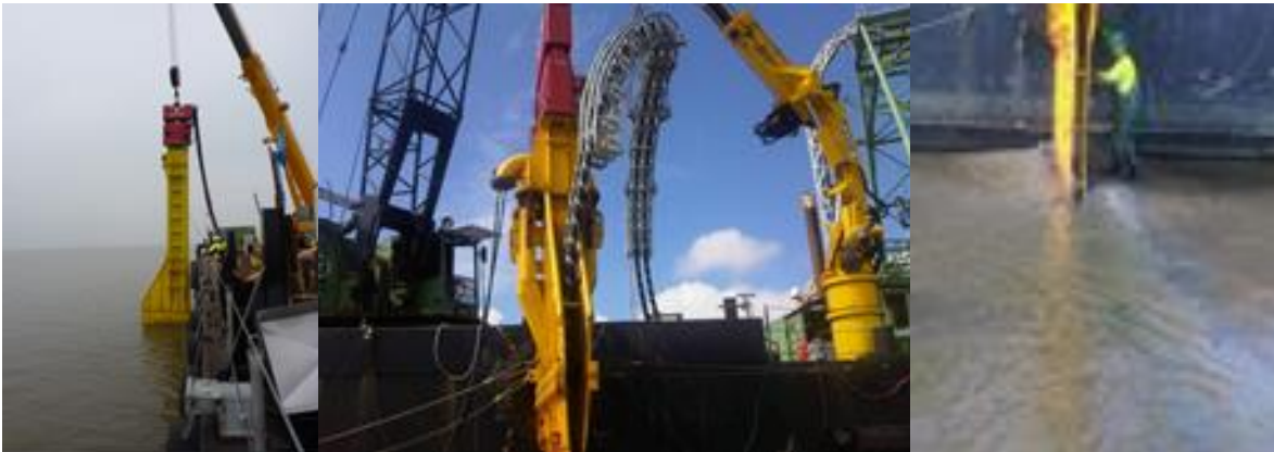
Figure 53 Vibration plough deployed from a barge
