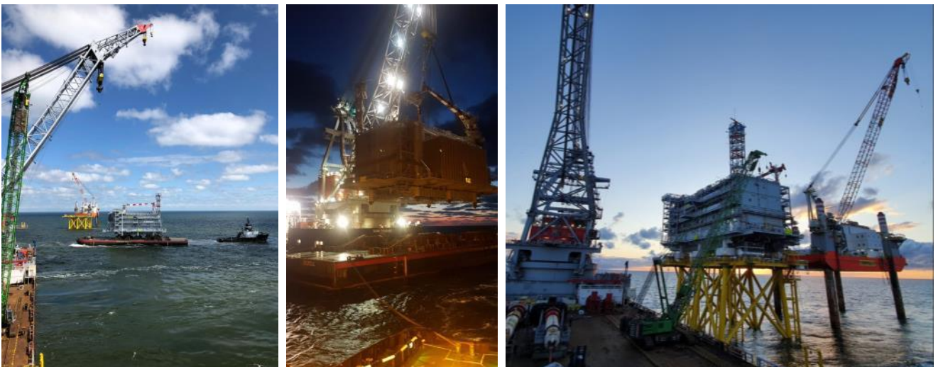
Figure 7a Installation of Borssele Alpha topside
