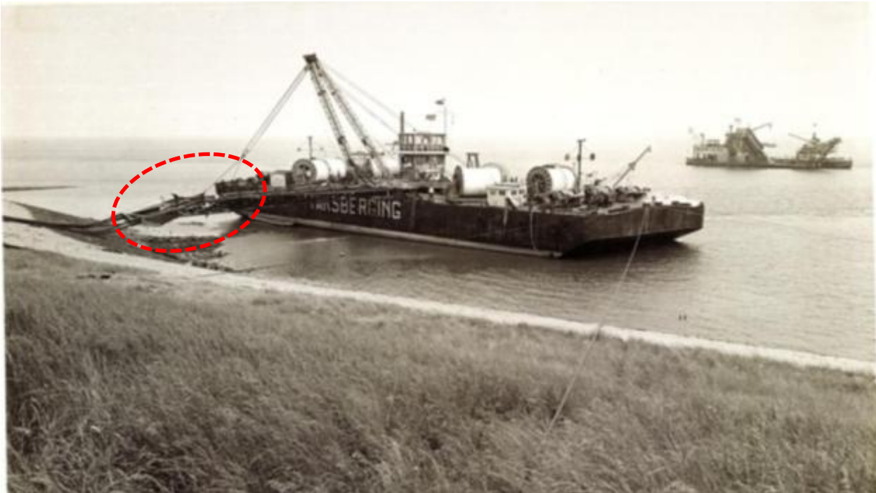
Figure 51 Cable installation by a vertical injector like trencher in Zeeland, location indicated in red
