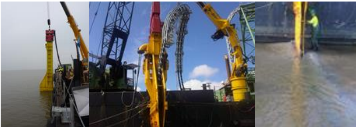
Figure 53 Vibration plough deployed from a barge
