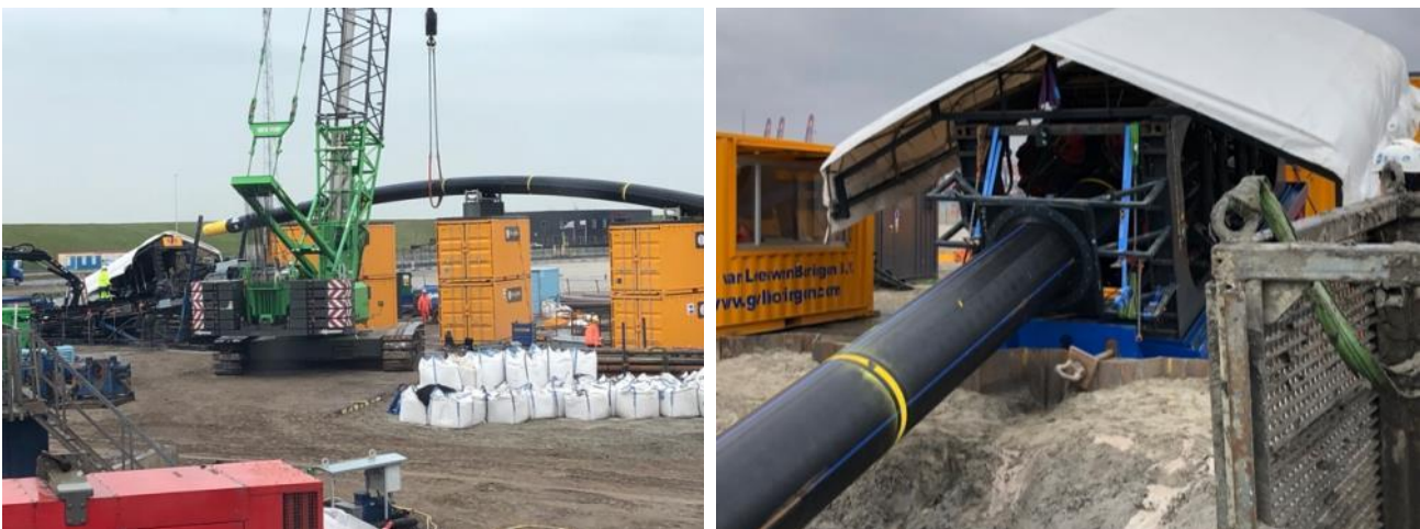
Figure 28 Pipe string supply into pipe pusher
