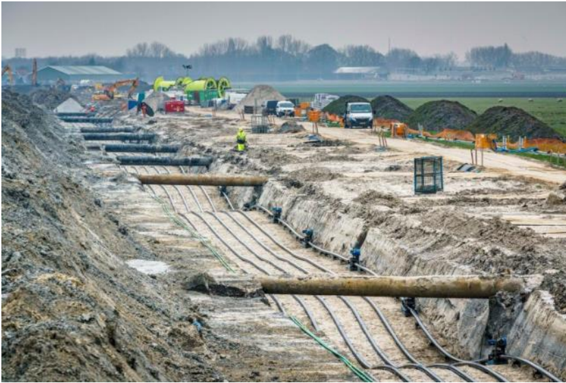
Figure 15 Example of a trench
