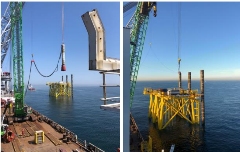
Figure 6 Pile driving at Borssele Alpha
