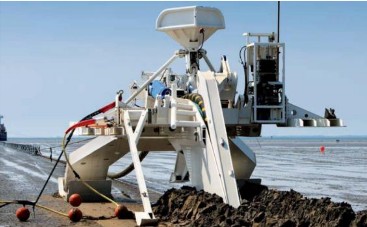
Figure 45 Sea Stallion cable plough
