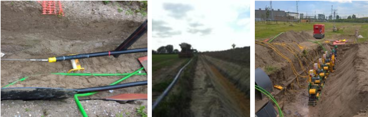
Figure 17 Pull in wire and rollers (left), backfilling before cable pull in (middle), typical roller (right)
