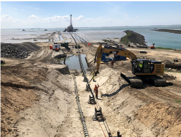
Figure 20 Cable pull in for project Borssele
