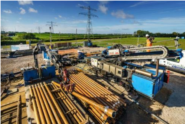
Figure 44 Example of HDD entry and exit point
