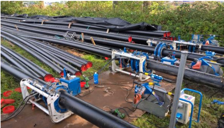
Figure 45 Welding of HDPE ducts
