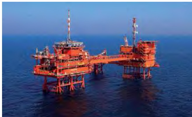
Figure 8.12: P15-ACD Processing & Accommodation Platforms. (Courtesy TAQA; TAQA, 2009)
