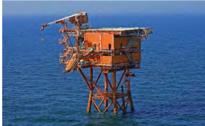
Figure 8.11: P18-A Satellite platform. (Courtesy TAQA; TAQA, 2009)
