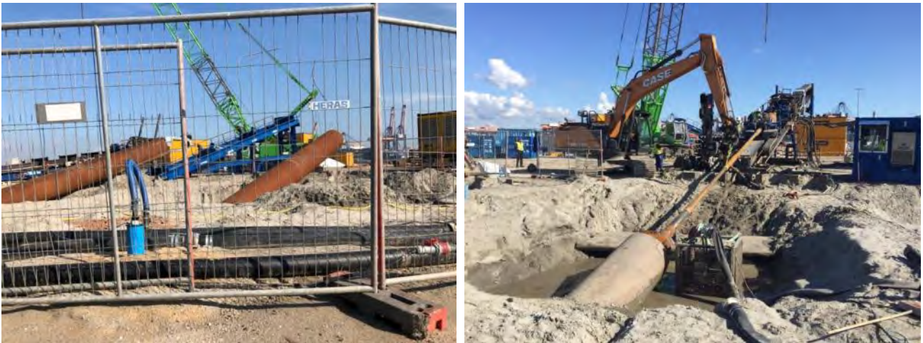
Figure 25 - Examples of reamer in HDDs
