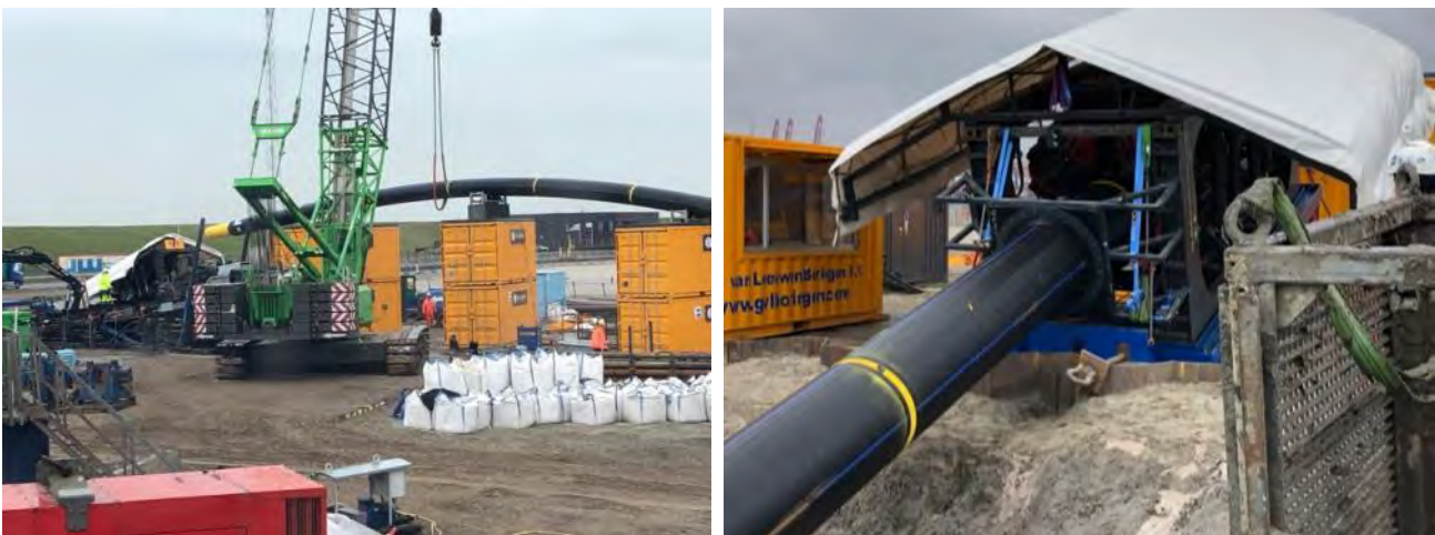
Figure 28 Pipe string supply into pipe pusher
