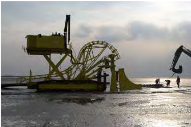
Figure 54 Vibration plough on tracks
