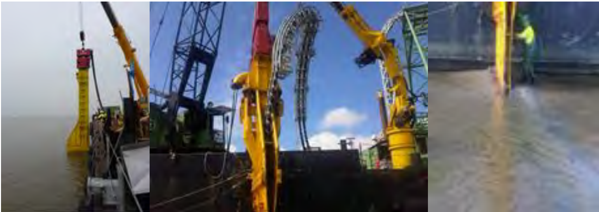
Figure 53 Vibration plough deployed from a barge
