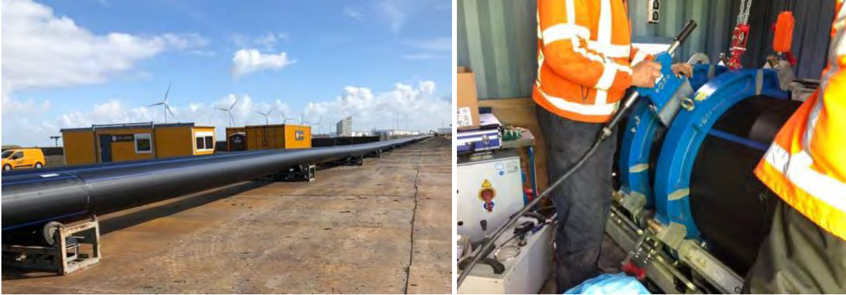
Figure 27 Pipe string assembly and mirror welding technique in container.
