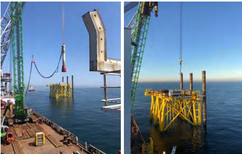
Figure 6 Pile driving at Borssele Alpha
