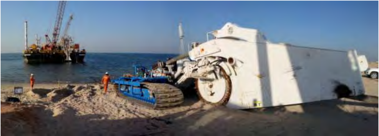
Figure 44 TM04 Wheel cutter cable trencher
