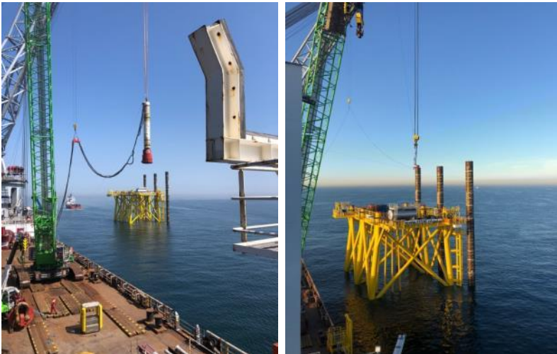
Figure 6 Pile driving at Borssele Alpha
