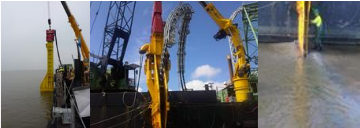
Figure 53 Vibration plough deployed from a barge
