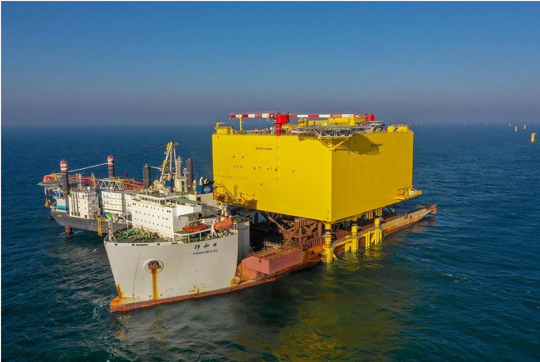
Figure 7b Float over installation of the BorWin3 topside in the German Bight
