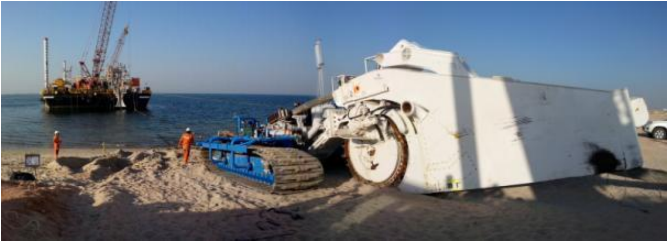
Figure 44 TM04 Wheel cutter cable trencher
