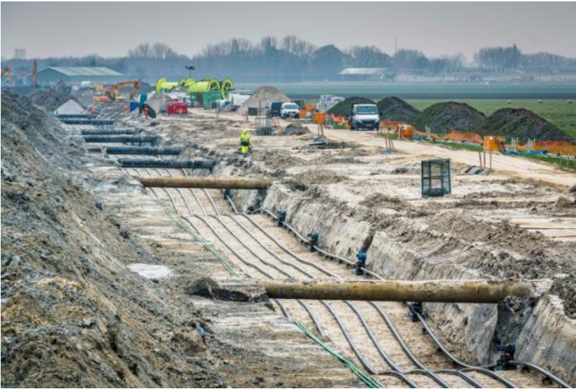
Figure 15 Example of a trench
