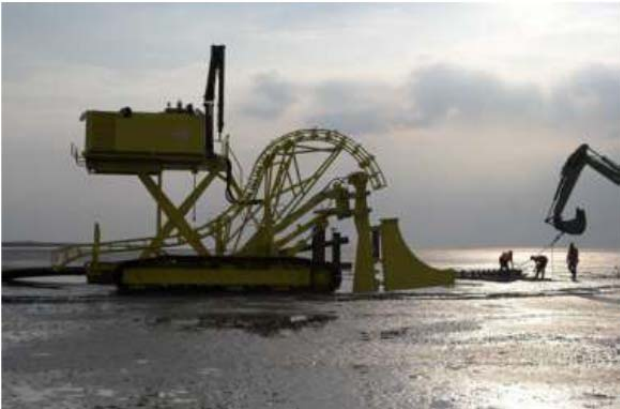
Figure 29 Vibration plough on tracks
