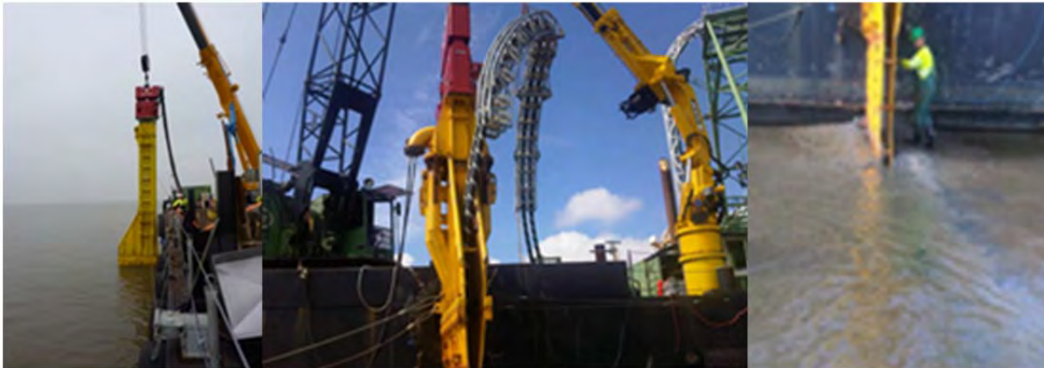
Figure 28 Vibration plough deployed from a barge
