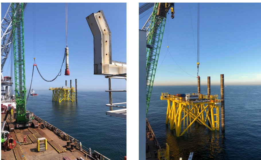
Figure 7 Piling of jacket
