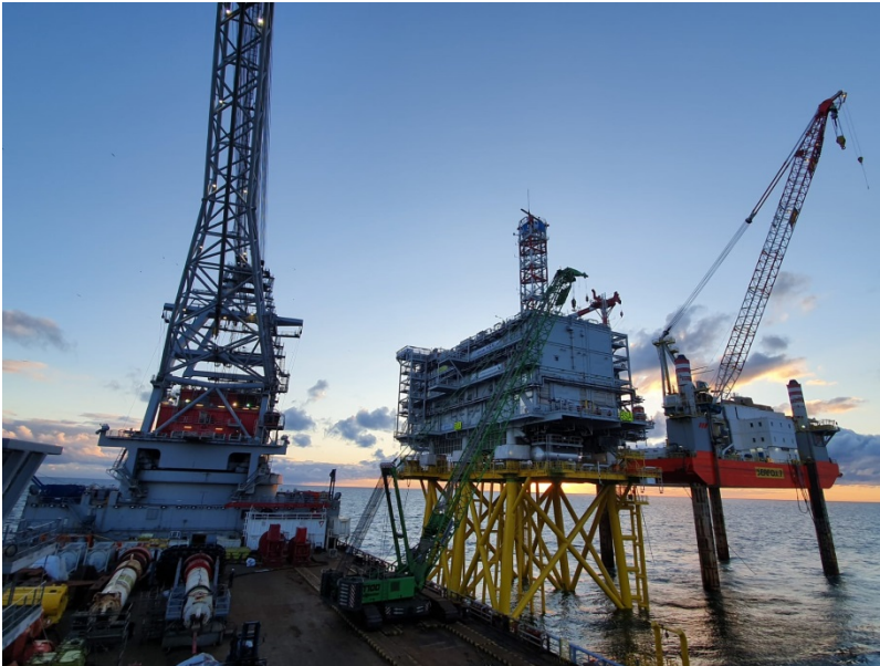
Figure 8 Installation of topside
