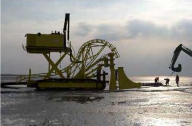
Figure 29 Vibration plough on tracks
