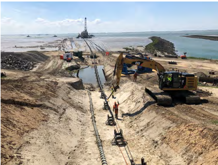
Figure 20 Cable pull in for project Borssele
