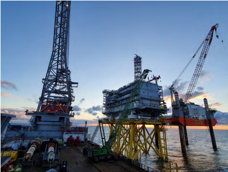
Figure 8 Installation of topside
