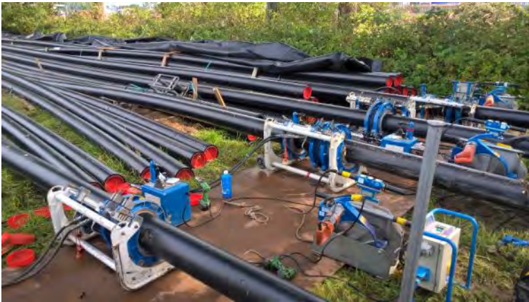
Figure 45 Welding of HDPE ducts
