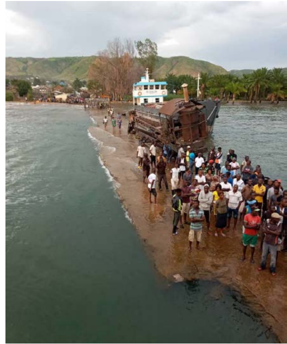
The Port of Moba has one pier. It is often partially submerged, due to the rising level of the lake. © Oscar Bahizi
