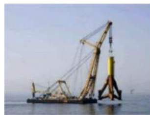
b) Shear-leg crane barge
