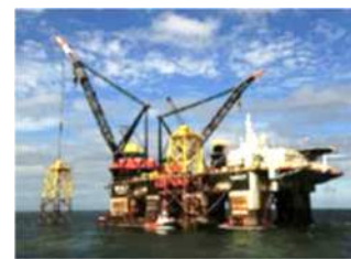
c) Semi-submersible heavy lift vessel
