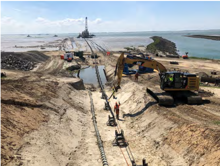
Figure 20 Cable pull in for project Borssele
