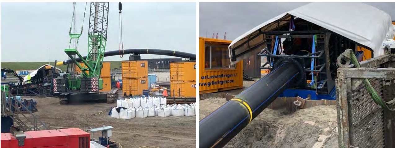
Figure 43 Pipe string supply into pipe pusher
