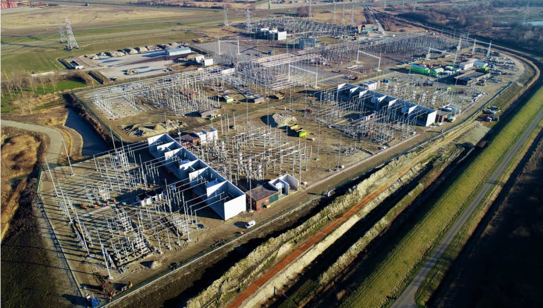
Figure 50 Transformer station Borssele during realisation
