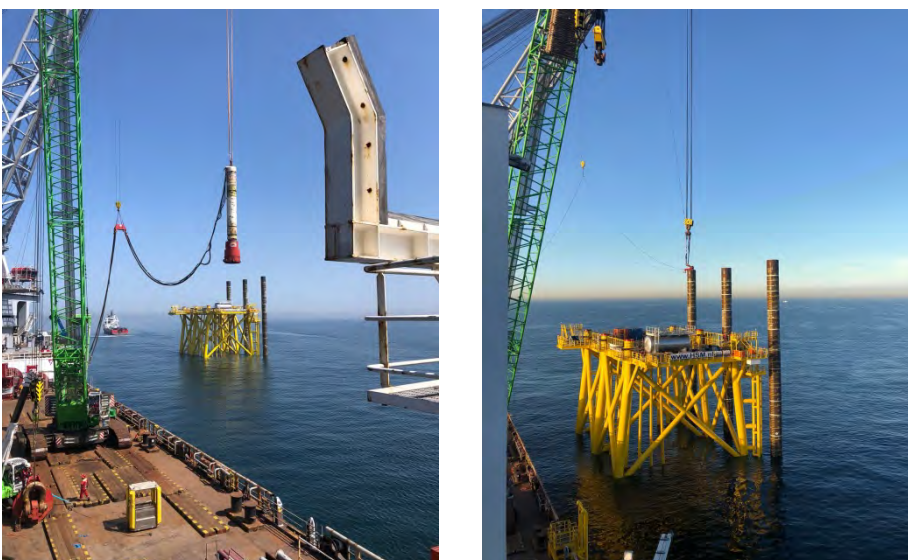
Figure 7 Piling of jacket
