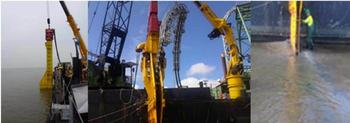
Figure 28 Vibration plough deployed from a barge
