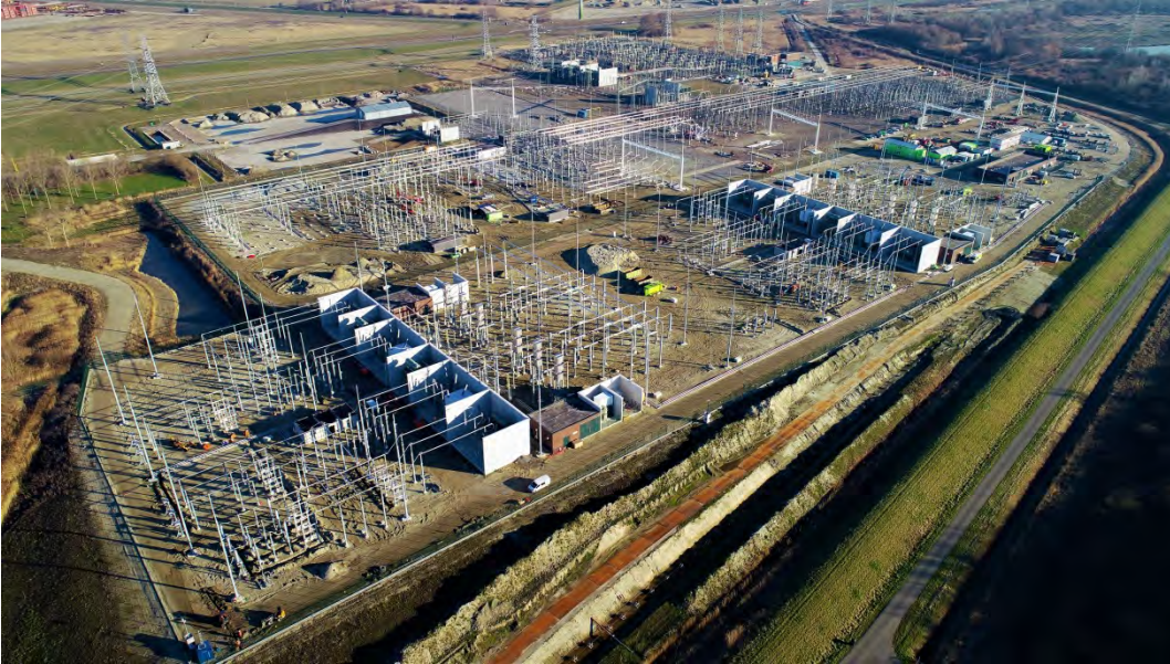
Figure 50 Transformer station Borssele during realisation
