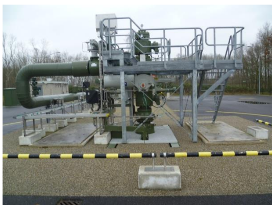
foto 1: Installatie / Well Head
