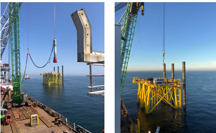
Figure 7 Piling of jacket
