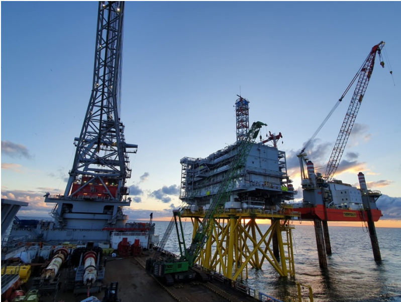
Figure 8 Installation of topside
