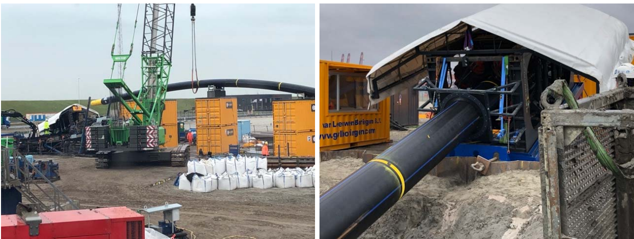
Figure 43 Pipe string supply into pipe pusher
