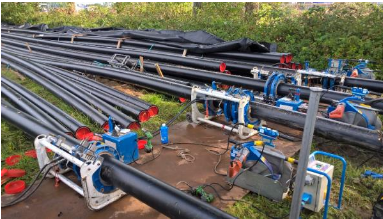
Figure 45 Welding of HDPE ducts
