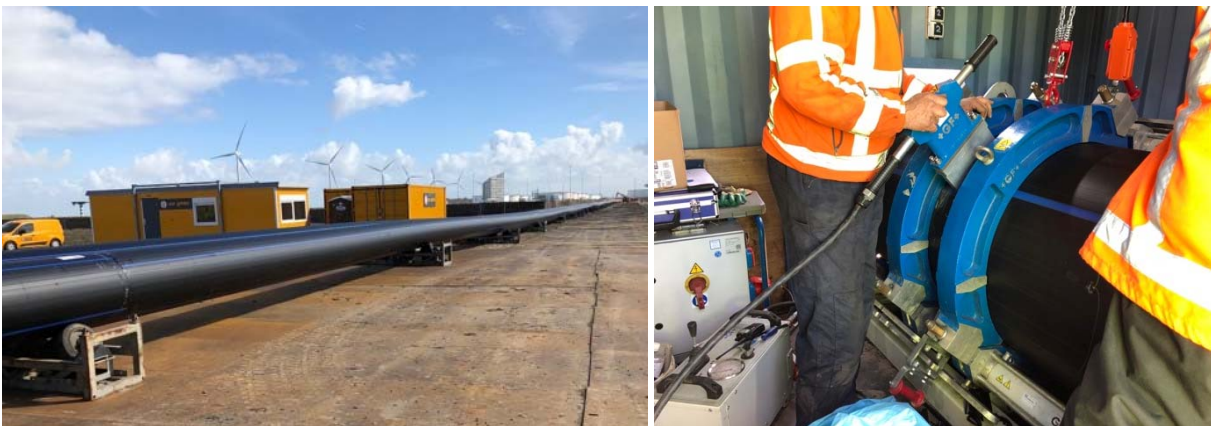
Figure 39 Pipe string assembly and mirror welding technique in container.
