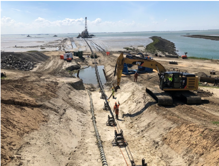
Figure 20 Cable pull in for project Borssele
