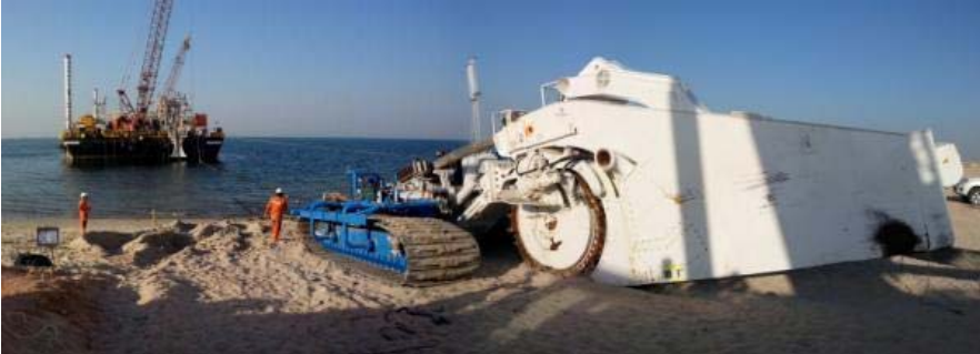
Figure 27 TM04 Wheel cutter cable trencher
