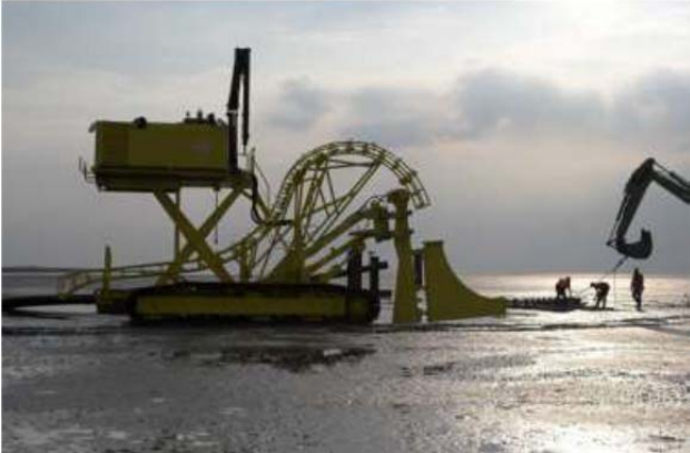
Figure 29 Vibration plough on tracks
