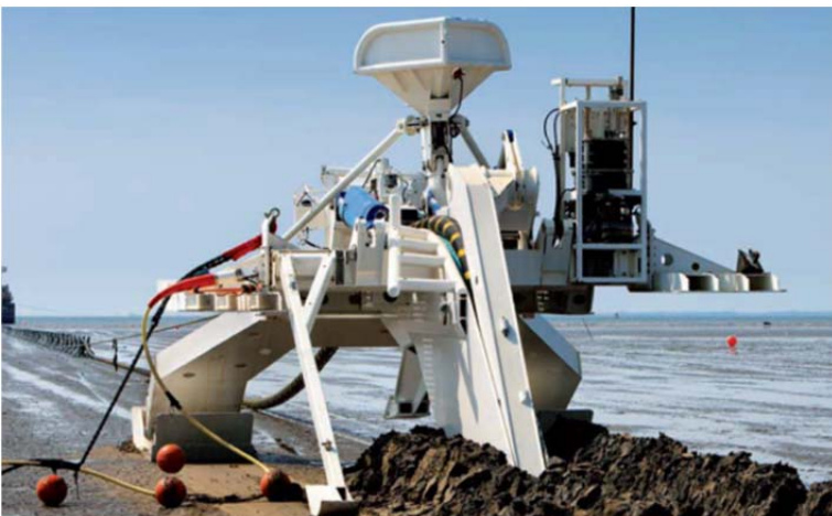
Figure 30 Sea Stallion cable plough
