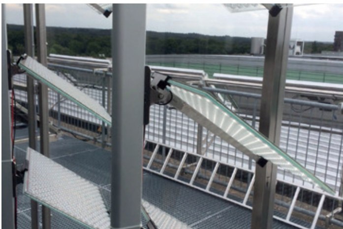
Wellsun's sun-tracking façade panels produce solar energy (with an efficiency of 30%), control natural lighting, act as a heat barrier and, at night-time, can be used as a media wall.
