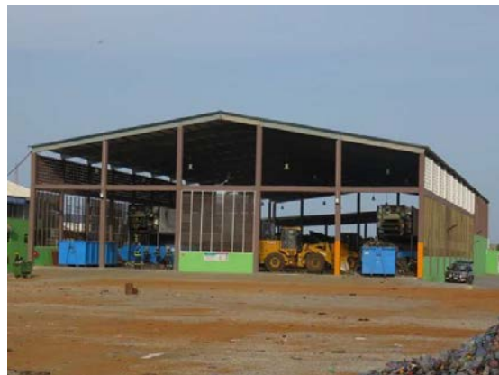
The facility is largely open air
