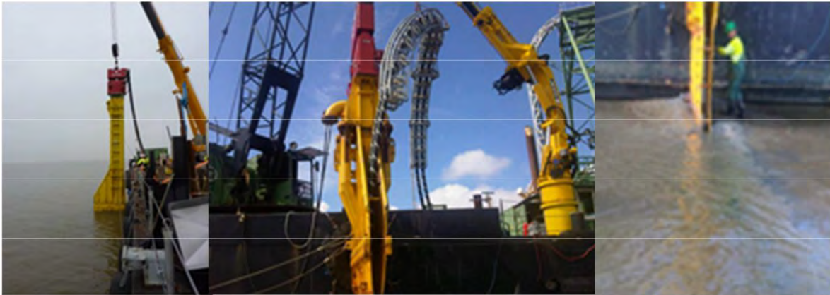
Figure 50 Vibration plough deployed from a barge
