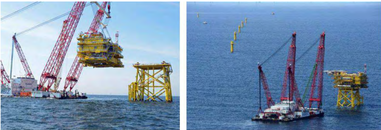
Figure 60 Installation of topside
