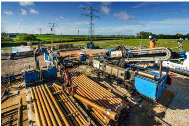
Figure 26 Example of HDD entry and exit point
