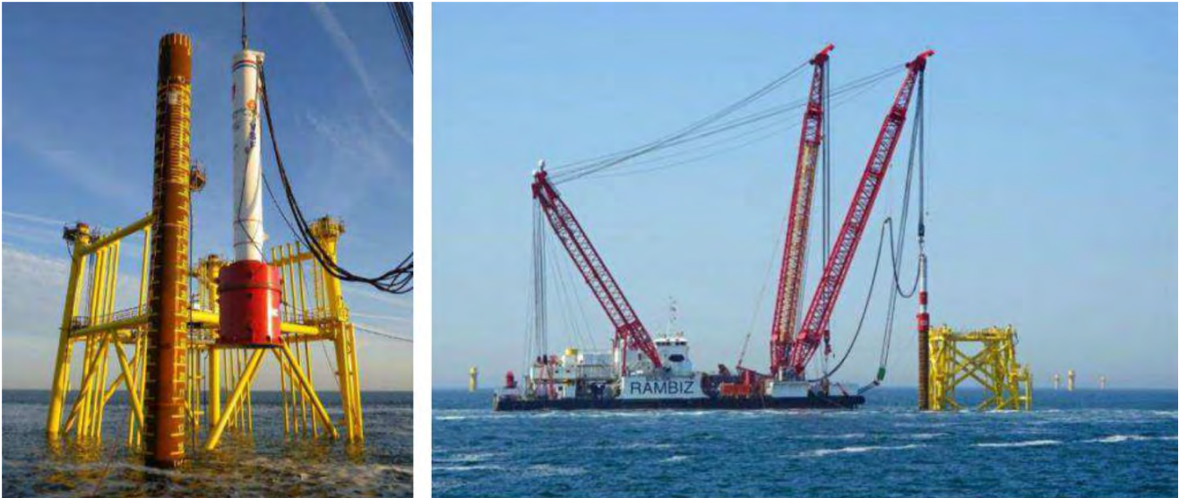
Figure 59 Piling of jacket
