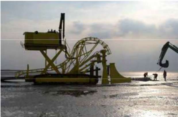
Figure 51 Vibration plough on tracks
