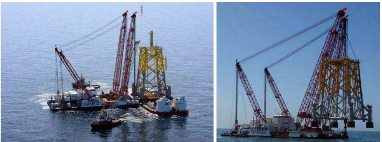
Figure 58 Installation of jacket
