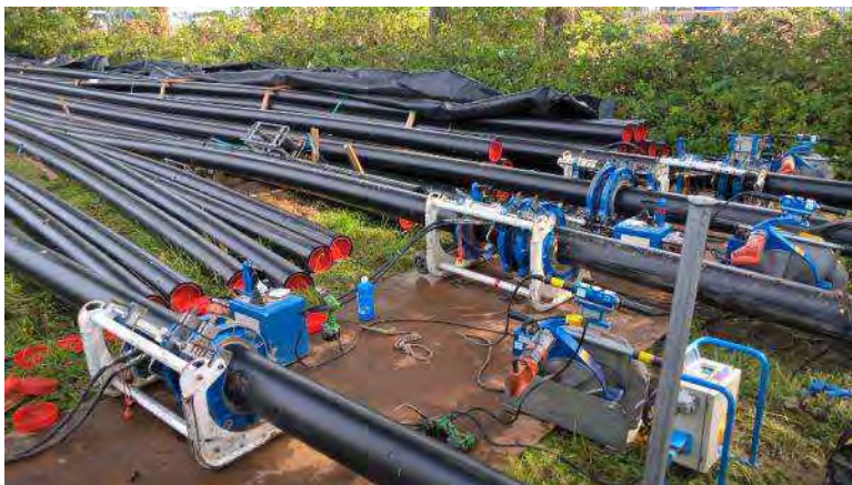
Figure 27 Welding of HDPE ducts
