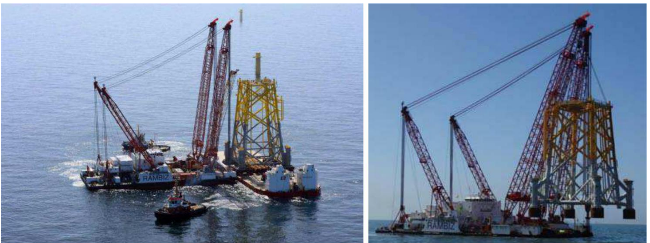
Figure 58 Installation of jacket
