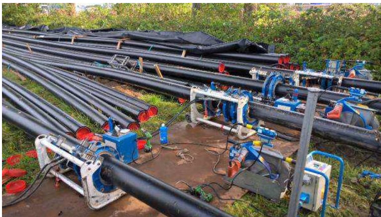
Figure 27 Welding of HDPE ducts
