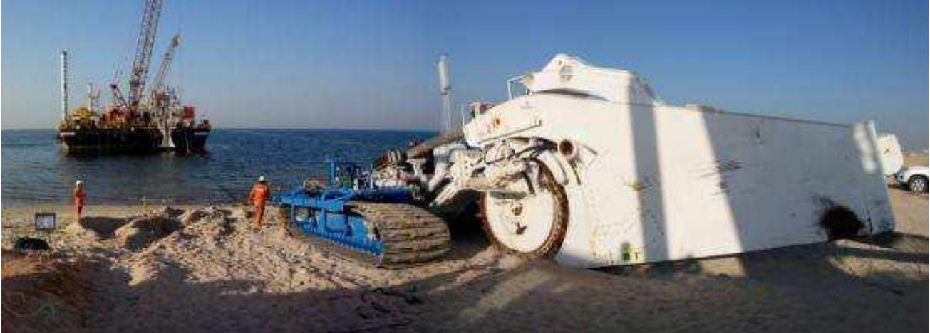
Figure 41 TM04 Wheel cutter cable trencher
