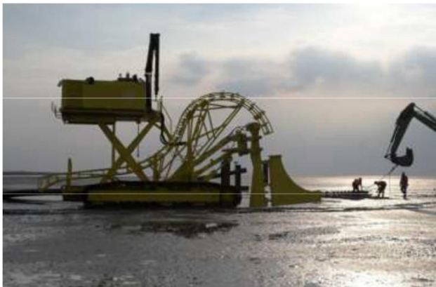
Figure 51 Vibration plough on tracks
