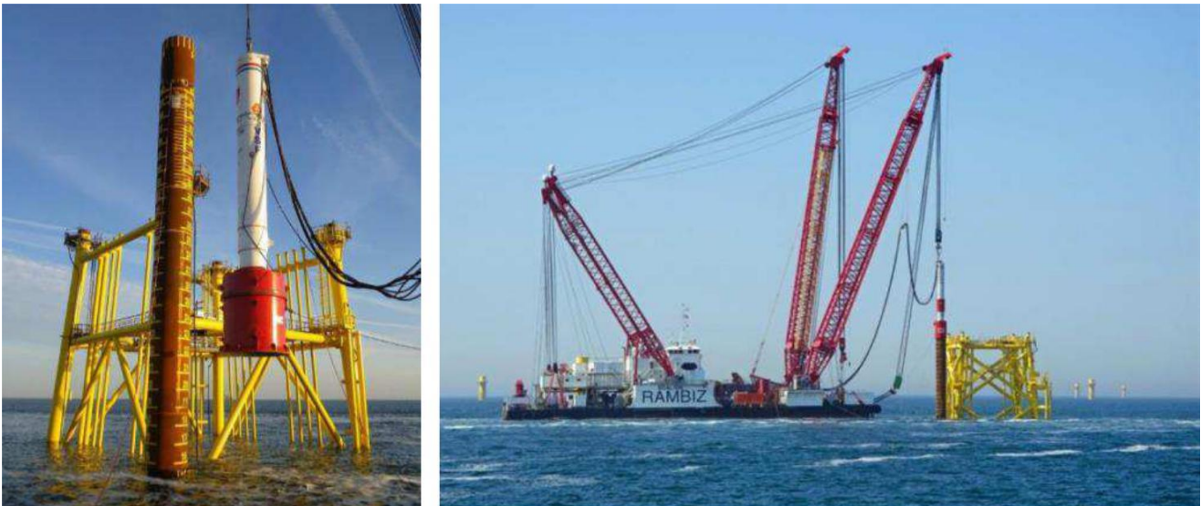
Figure 59 Piling of jacket
