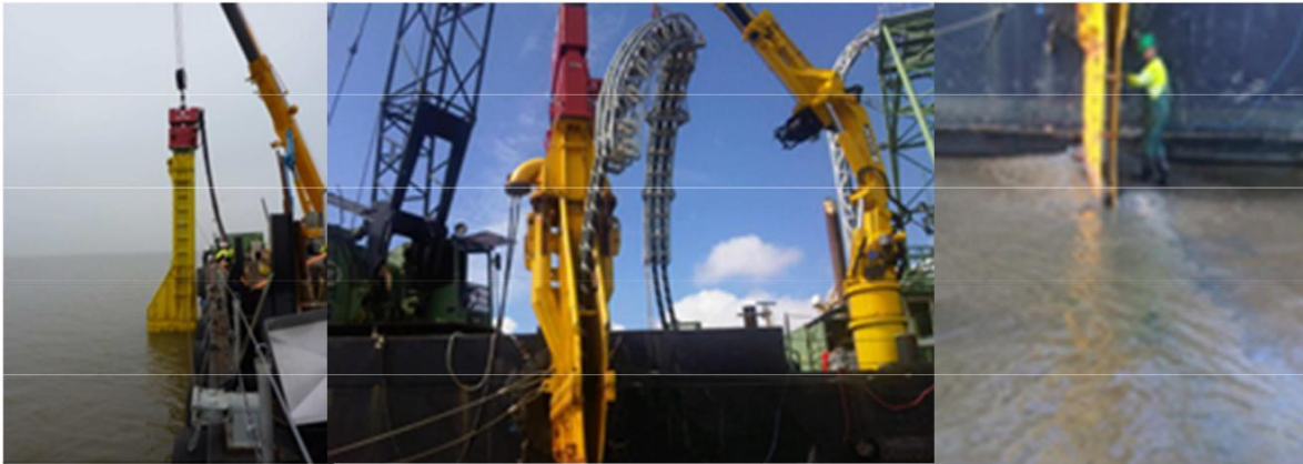
Figure 50 Vibration plough deployed from a barge
