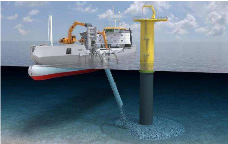
Figure 57 Rock installation vessel
