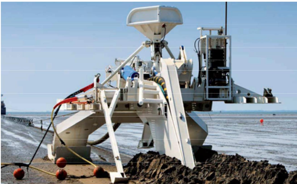
Figure 42 Sea Stallion cable plough
