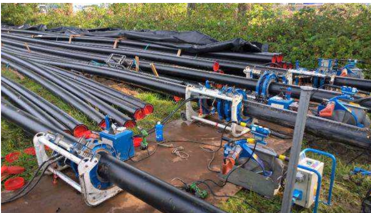
Figure 27 Welding of HDPE ducts
