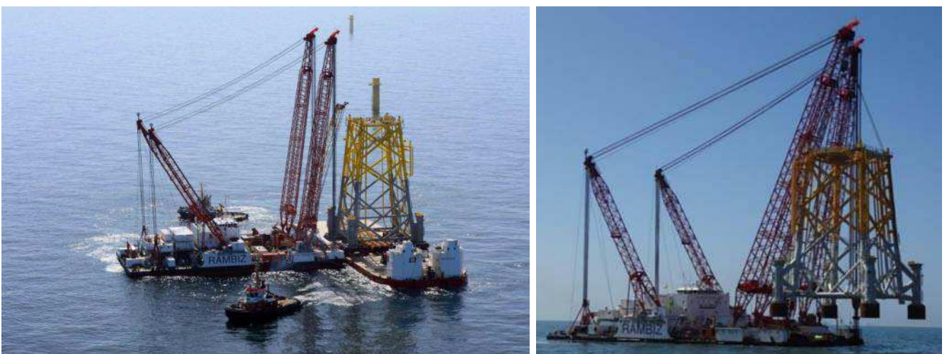
Figure 58 Installation of jacket
