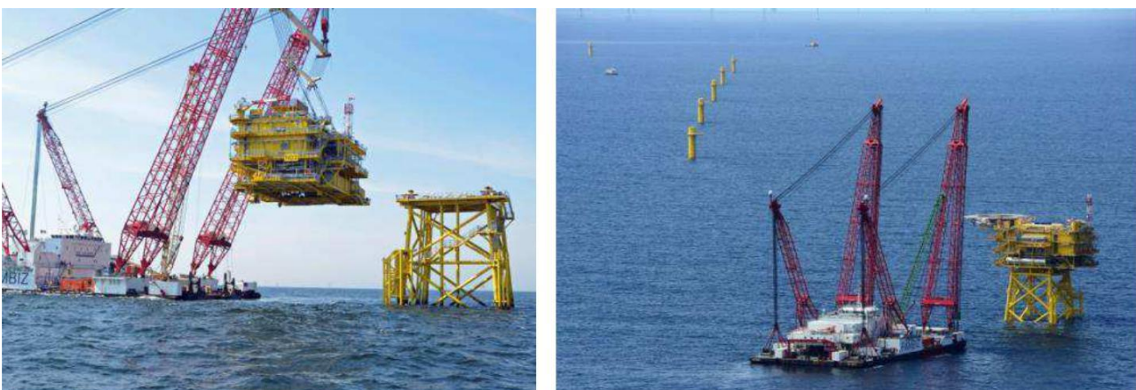
Figure 60 Installation of topside
