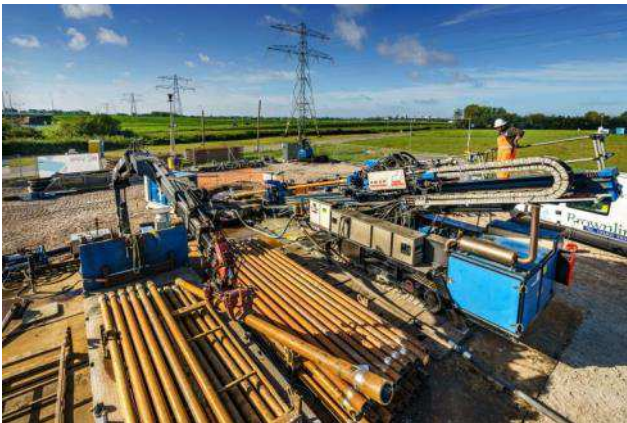
Figure 26 Example of HDD entry and exit point
