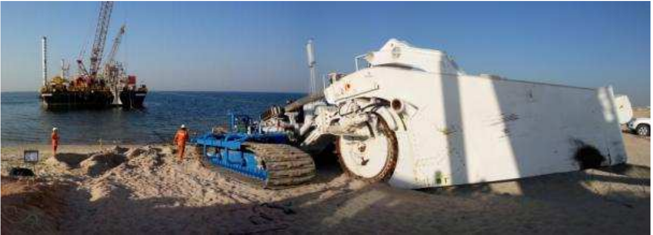
Figure 41 TM04 Wheel cutter cable trencher
