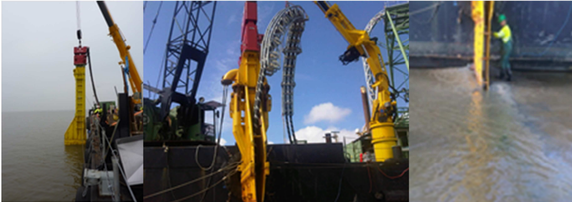
Figure 50 Vibration plough deployed from a barge
