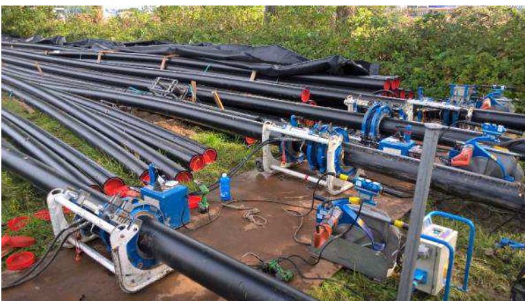
Figure 27 Welding of HDPE ducts
