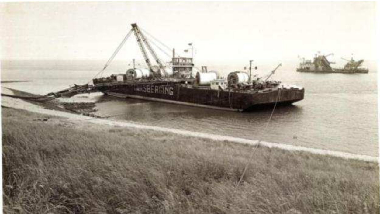
Figure 48 Cable installation by a vertical injector like trencher in Zeeland
