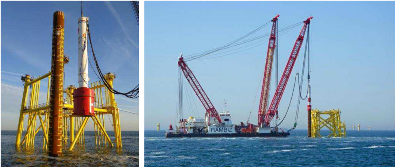
Figure 59 Piling of jacket
