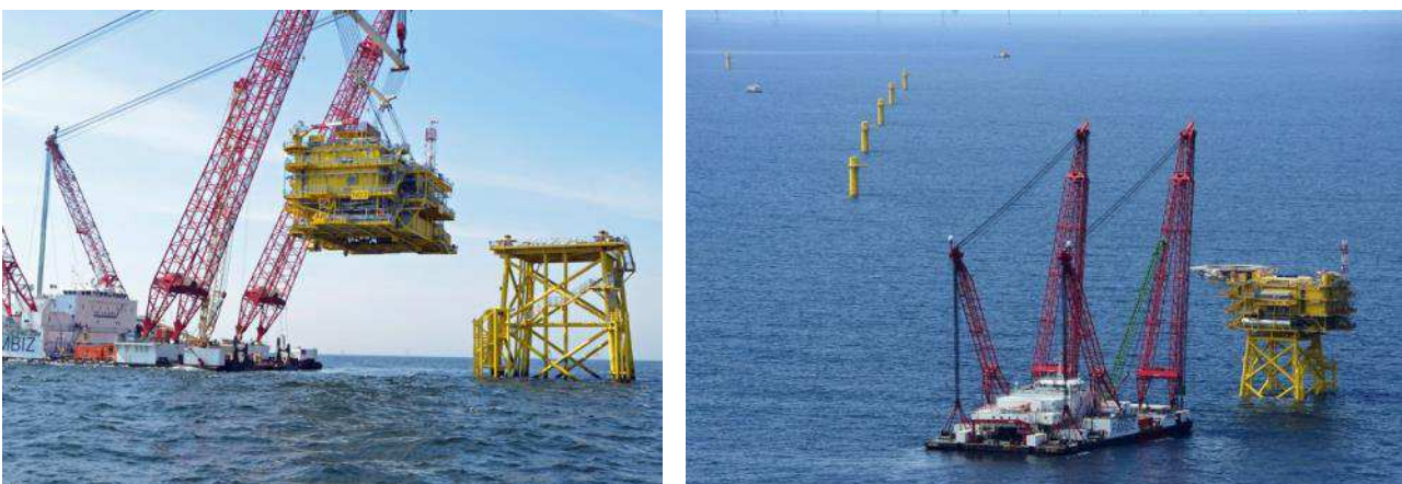
Figure 60 Installation of topside
