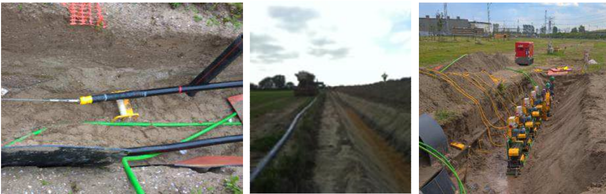
Figure 16 Pull in wire and rollers (left), backfilling before cable pull in (middle), typical roller (right)
