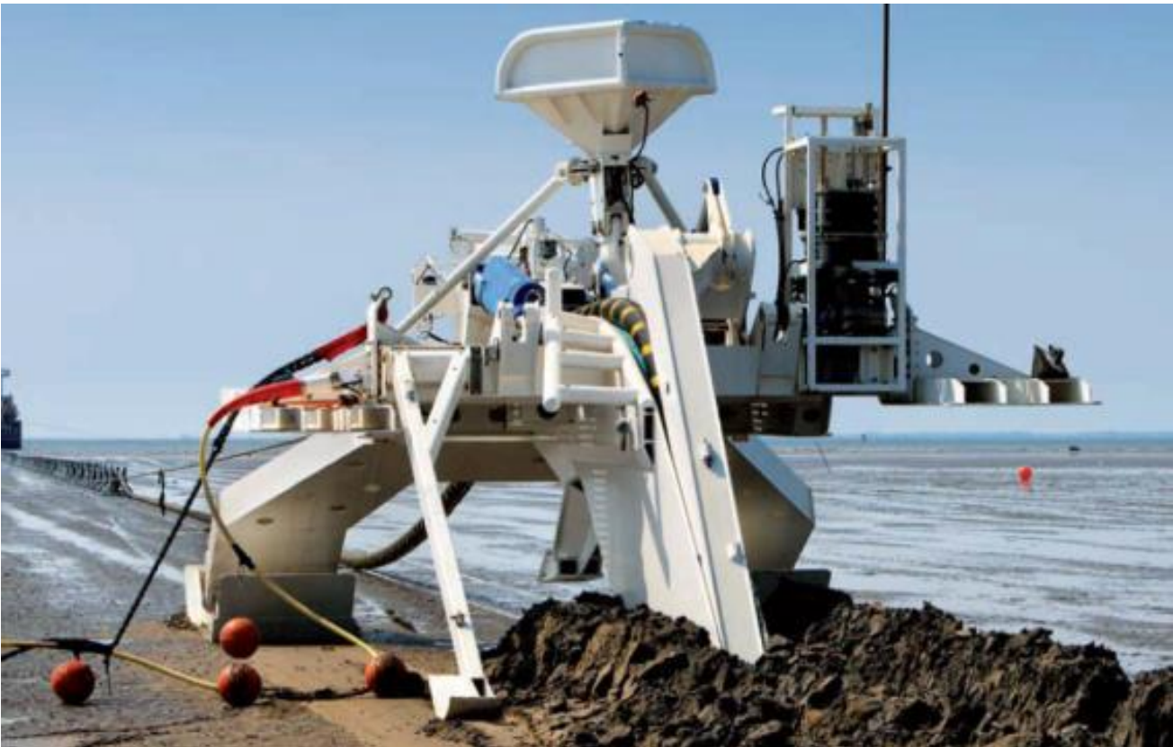
Figure 25 Sea Stallion cable plough
