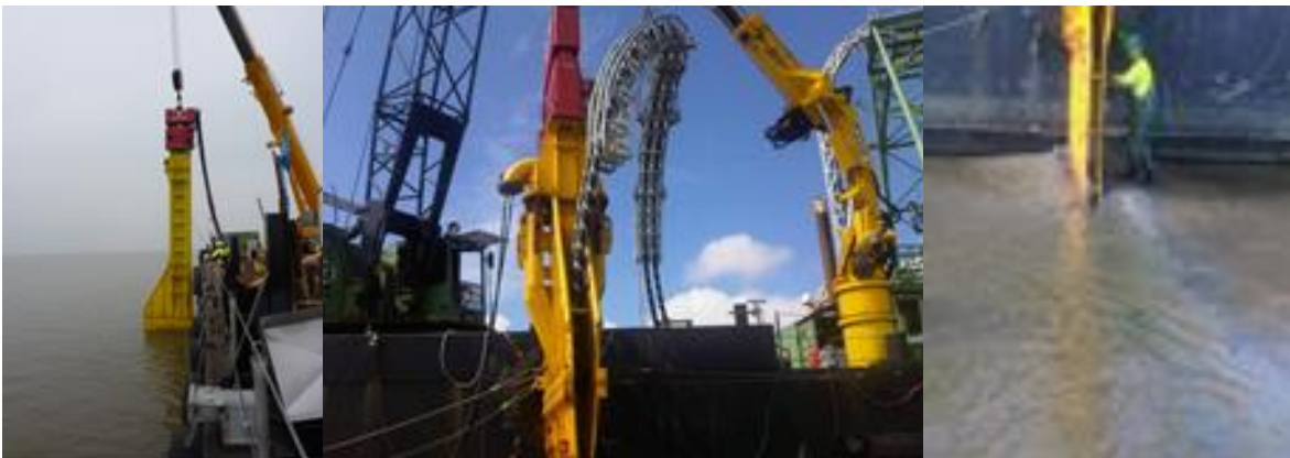
Figure 51 Vibration plough deployed from a barge
