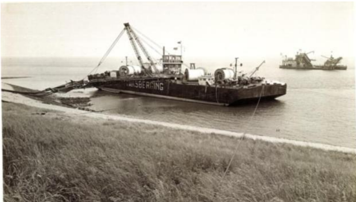
Figure 49 Cable installation by a vertical injector like trencher in Zeeland
