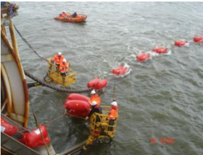
Figure 23 Attaching of floatation on the cable
