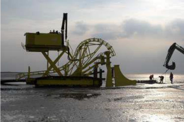
Figure 52 Vibration plough on tracks
