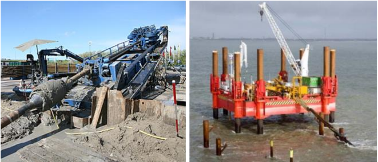
Figure 33 (left) Drilling installation - (right) Jack up barge with a drilling installation
