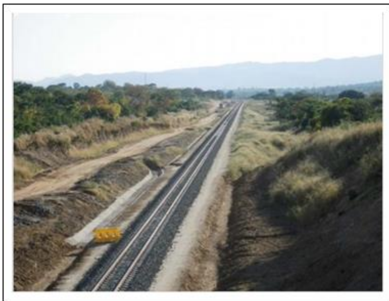
Figure 8: part of new mono-railway in Malawi between Tete and Nacala ( http://www.mkango.ca/s/photogallery.asp?send=now&ReportID=453005 )
