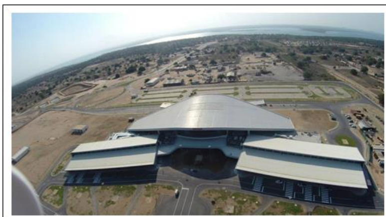
Figure 11: Nacala international airport ( http://www.clubofmozambique.com/solutions1/sectionnews.php?secao=mozambique&id=2147485968&tipo=one )
