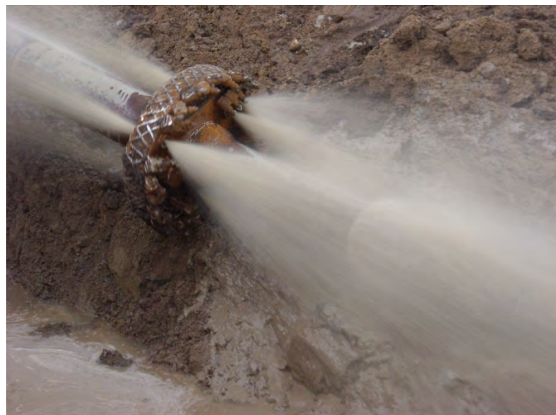
Bentoniet flushing out of the nozzles of the fly cutter
